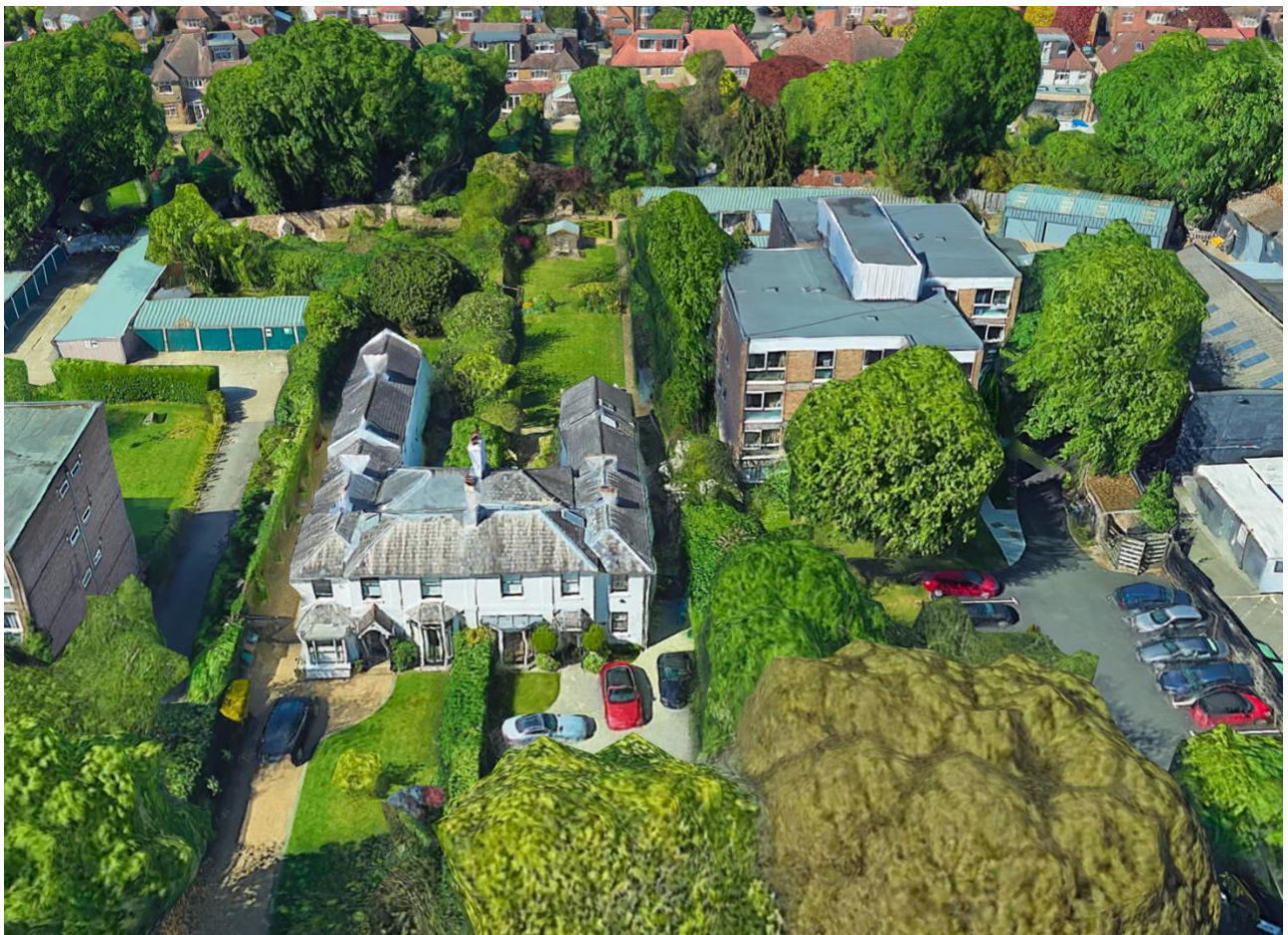
Fig. 16: Birdseye view of the grade II listed Albion Cottage/Albion Lodge © Google Earth, which are not easily seen from street level owing to mature boundary treatments/screening. The flat roofs of the garages currently on the Site are just visible behind (north of) Lynton Grange, to the east of the listed building).
