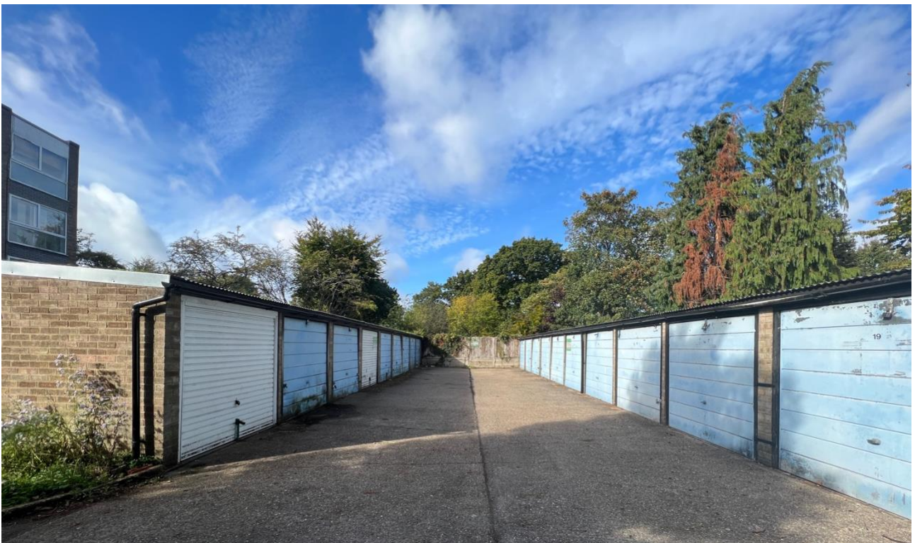
Fig. 13: Both rows of garages with Lynton Grange apartment block visible far left.
