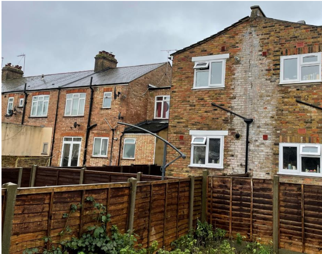
Figure 2 – The rear elevation of the site with No. 31
