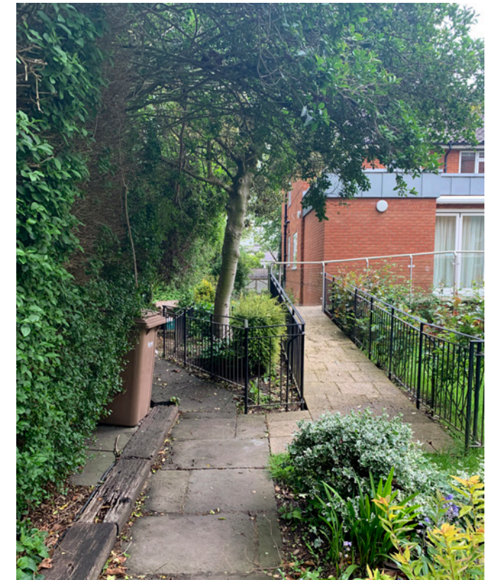
Existing ramped access to extension building.
