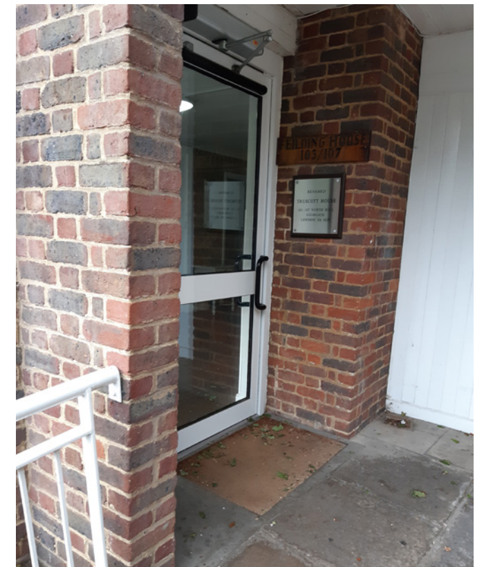
Existing main entrance at Truscott House.
