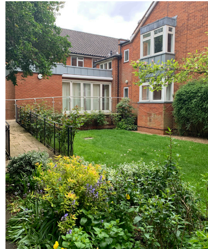
Unsympathetic extension to Kekewich House.
