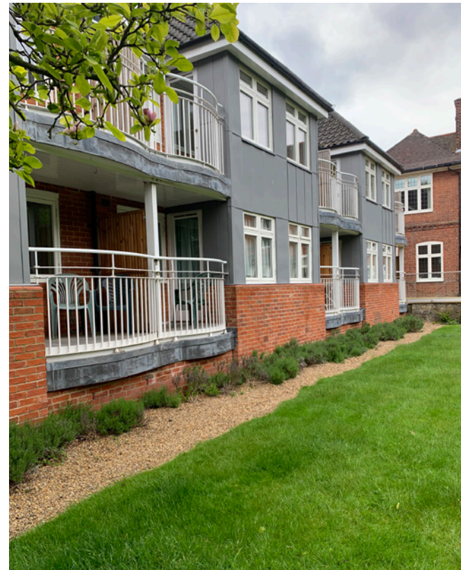
Contemporary extension building at rear garden.
