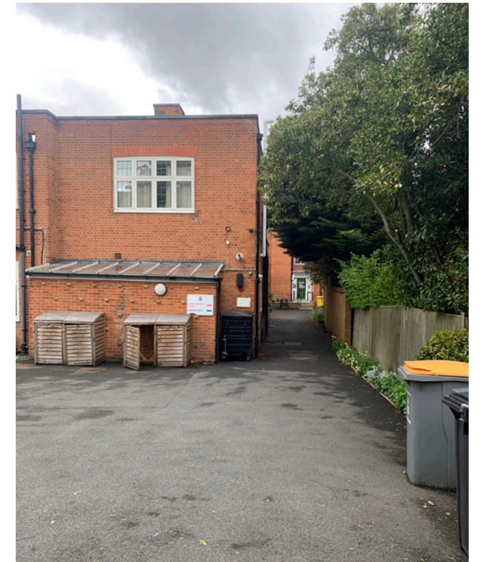
Unsympathetic extension to Kekewich House.
