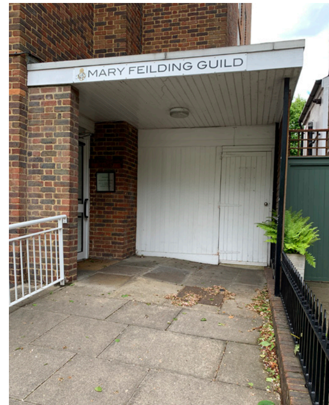
Existing main entrance at Truscott House.
