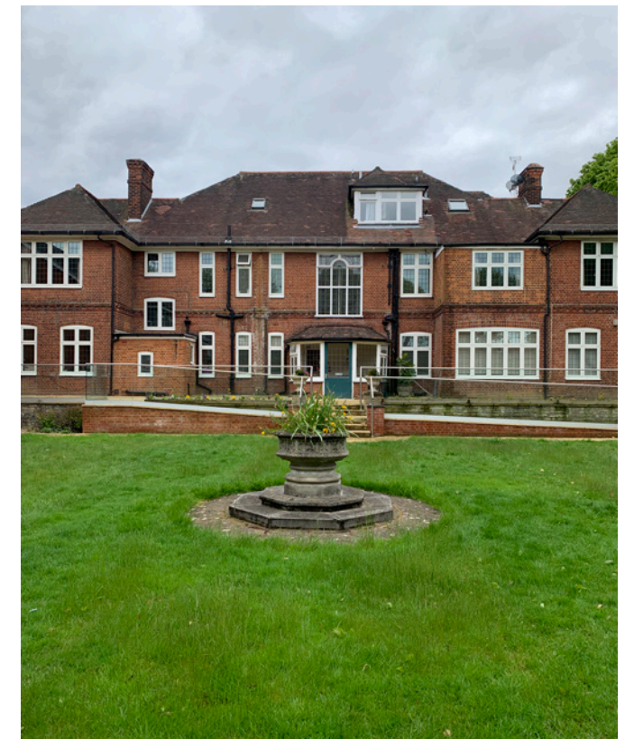
Rear of Kekewich House.
