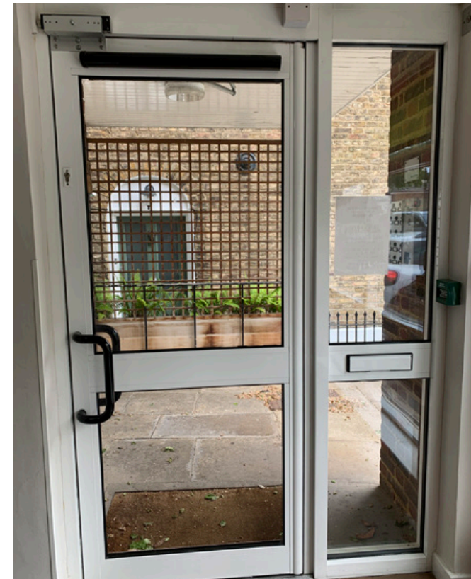
Existing Main entrance door with aspect overlooking 109 North Hill entrance.
