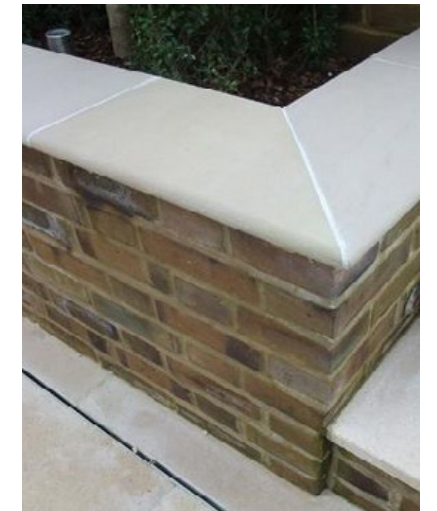
Low level walls enclose the basement lightwell (no walling to the site frontage).
