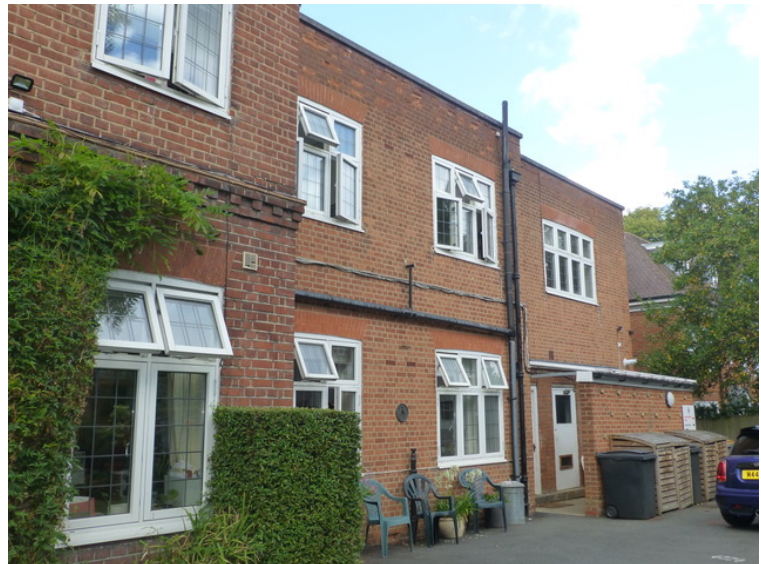
Figure 7: The eastern extension on View Road
