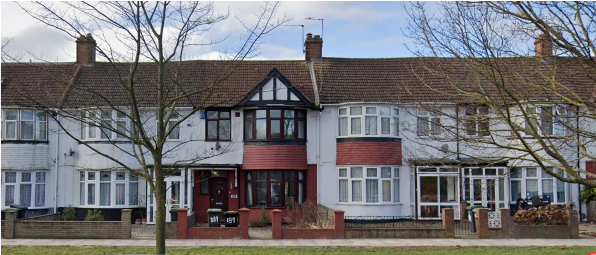
Exisitng Street View
