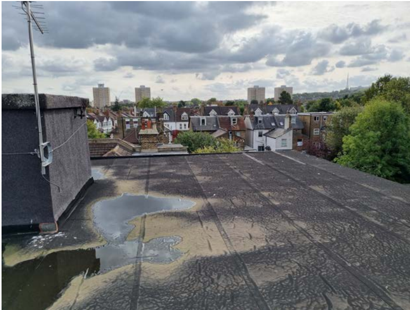
View towards south from the roof of Palm Court
