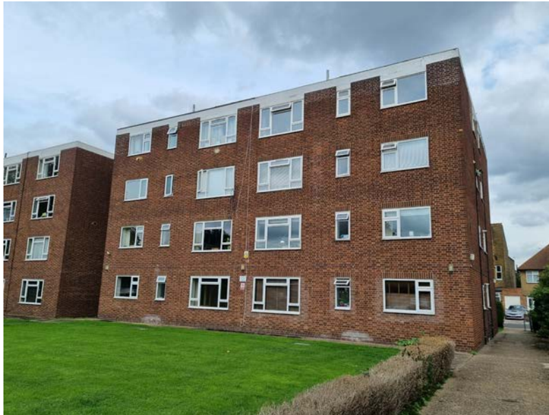
Rear view of Palm Court
