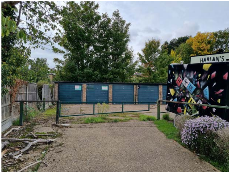
View of the garages in the rear garden
