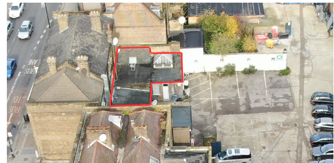
Figure 10: Rear Buildings of 804-806 High Road
