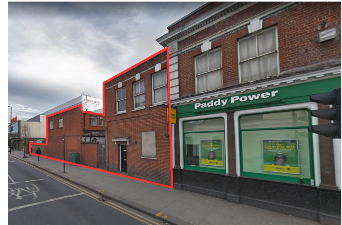
Figure 9: Rear Buildings of 814 High Road
