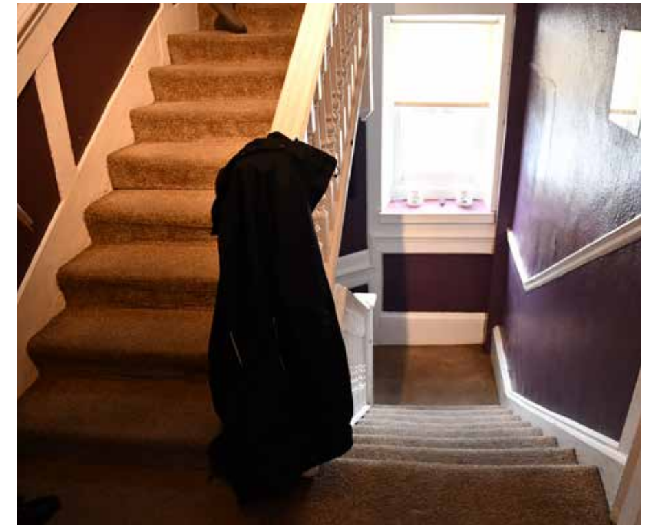
FIGURE 40. No. 808 existing first floor staircase
