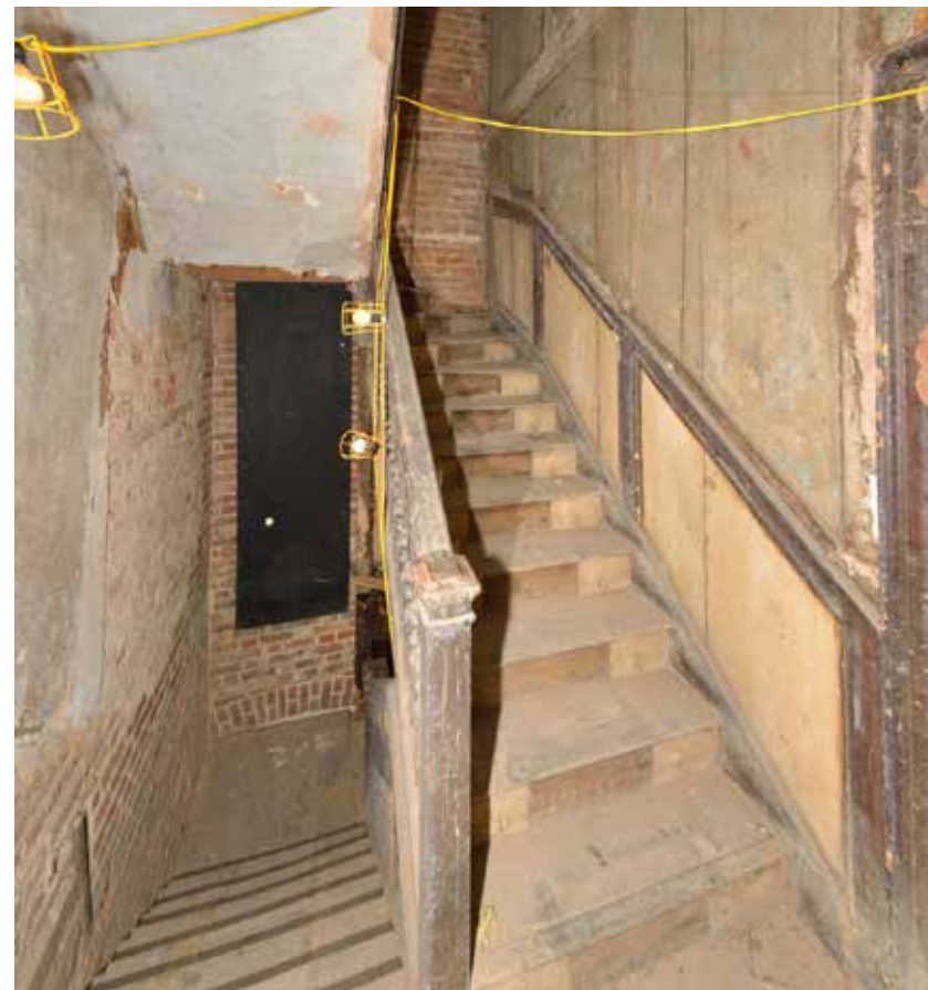
FIGURE 37. No. 810/12 existing first floor staircase
