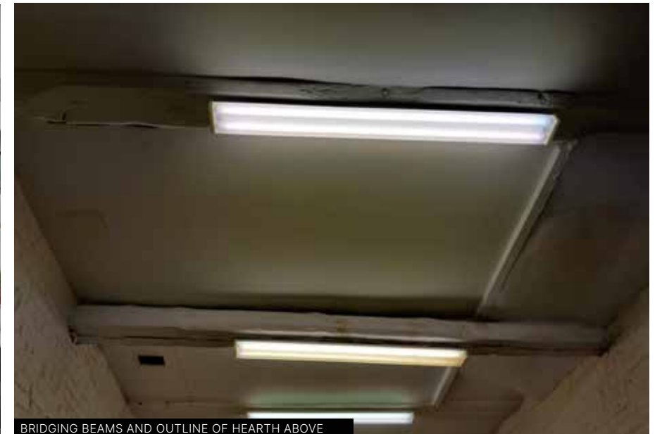
BRIDGING BEAMS AND OUTLINE OF HEARTH ABOVE
