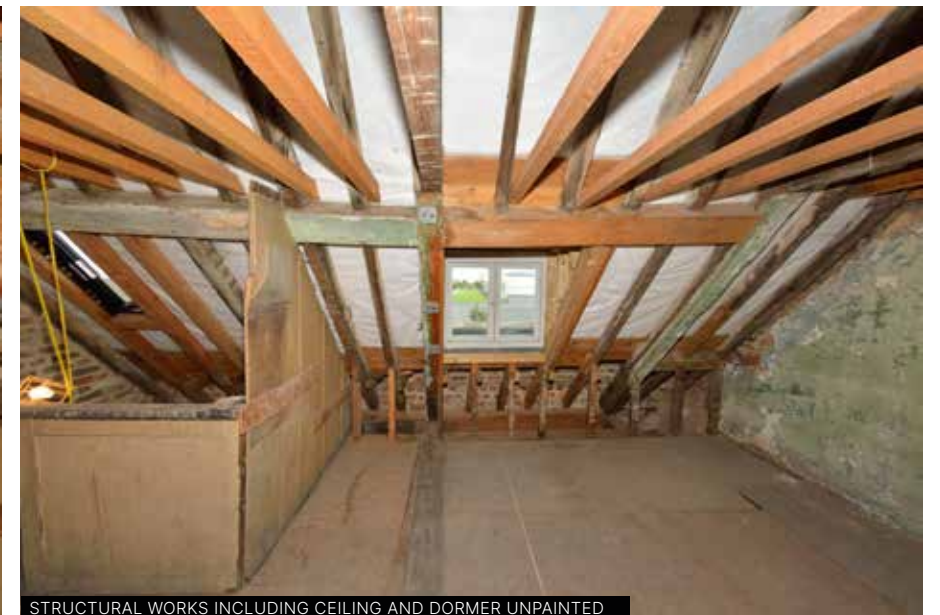
STRUCTURAL WORKS INCLUDING CEILING AND DORMER UNPAINTED
