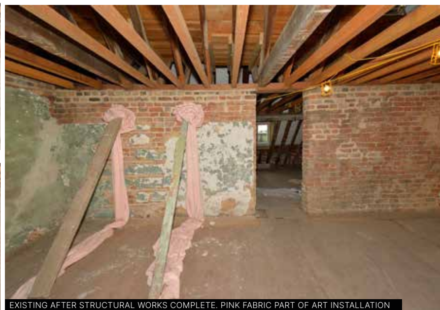
EXISTING AFTER STRUCTURAL WORKS COMPLETE. PINK FABRIC PART OF ART INSTALLATION
