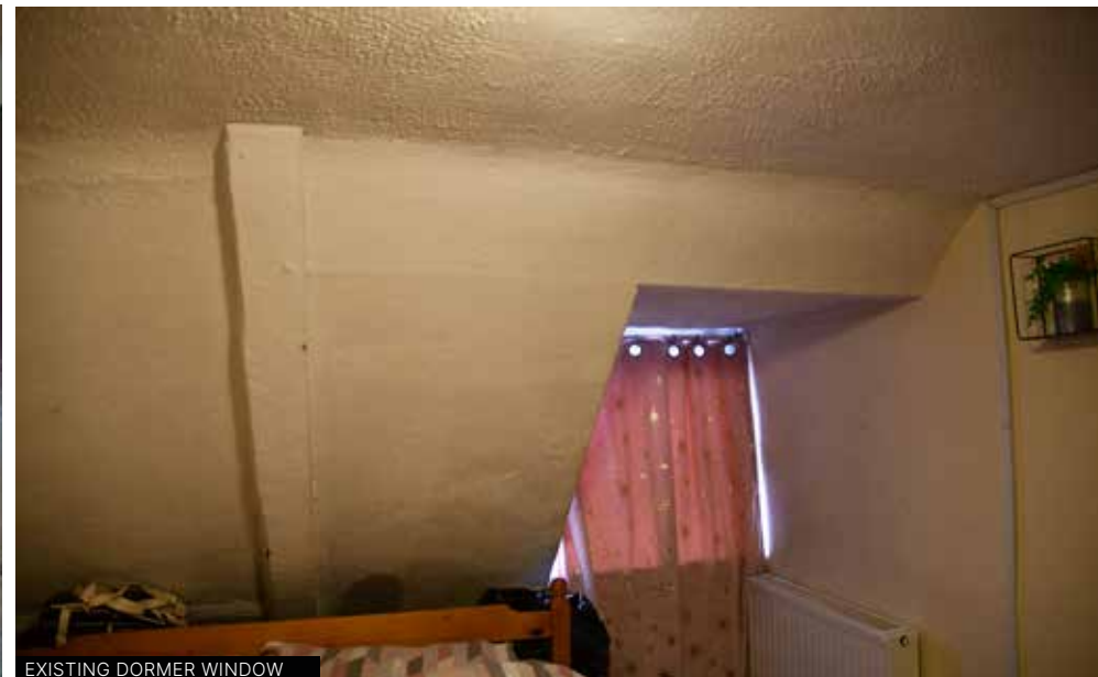
EXISTING DORMER WINDOW
