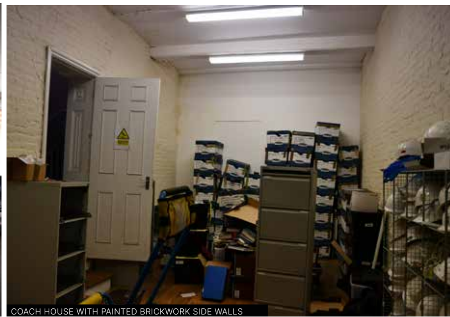
COACH HOUSE WITH PAINTED BRICKWORK SIDE WALLS
