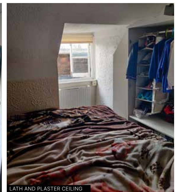
LATH AND PLASTER CEILING
