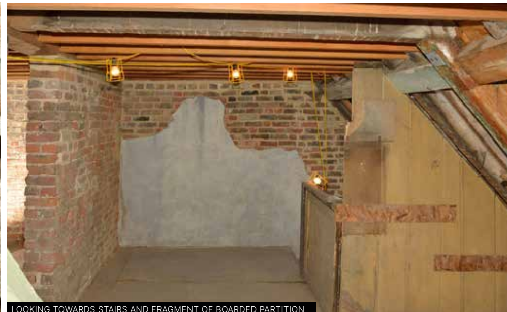
LOOKING TOWARDS STAIRS AND FRAGMENT OF BOARDED PARTITION
