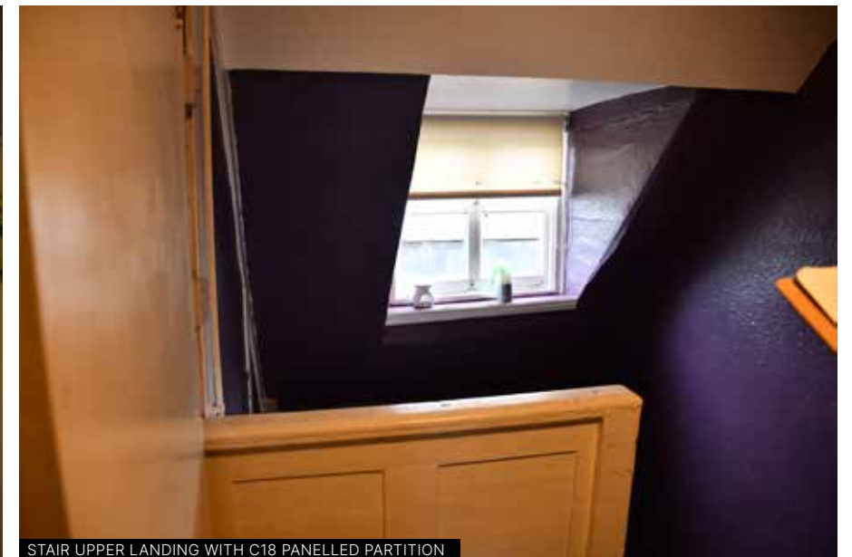
STAIR UPPER LANDING WITH C18 PANELLED PARTITION
