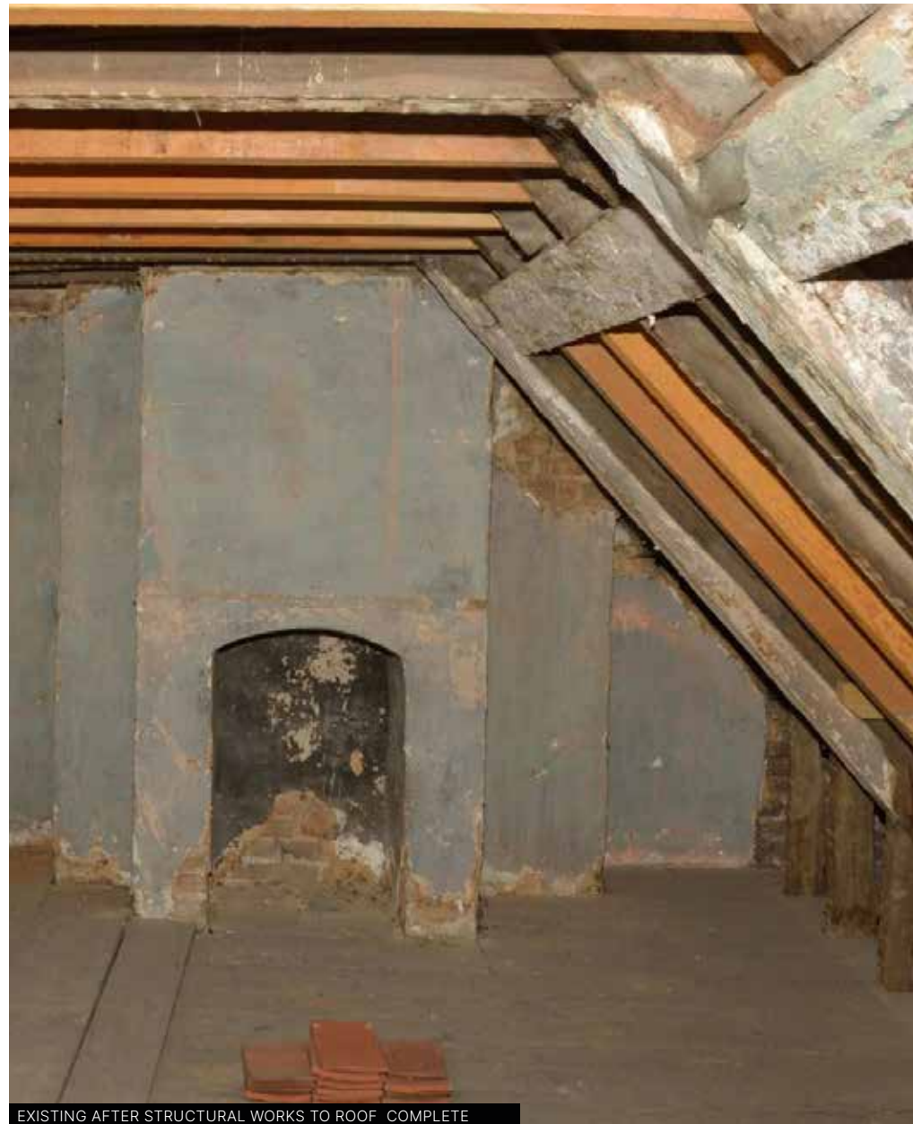
EXISTING AFTER STRUCTURAL WORKS TO ROOF COMPLETE
