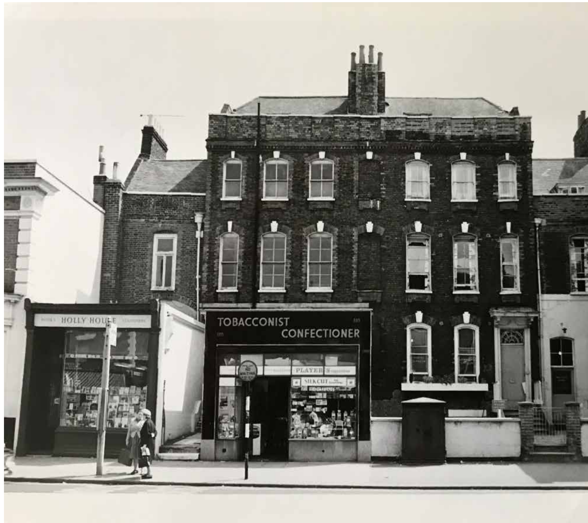
FIGURE 20. Street elevation of 808-810/812, 1980
