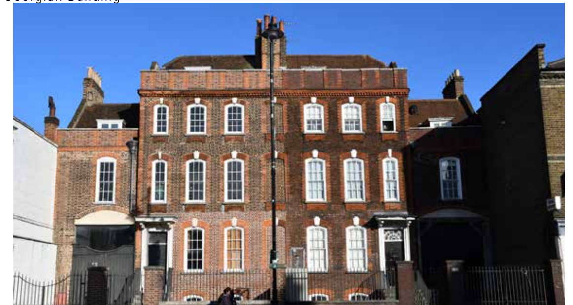
FIGURE 8. Street elevation of 808-810/812
