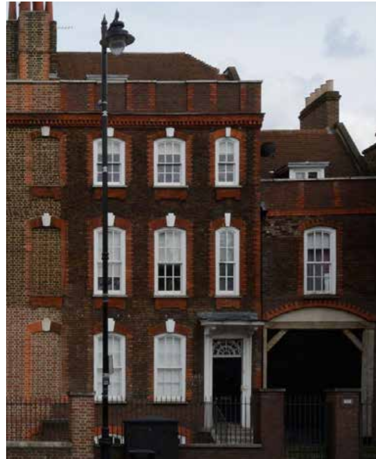
FIGURE 9. Street elevation of 808
