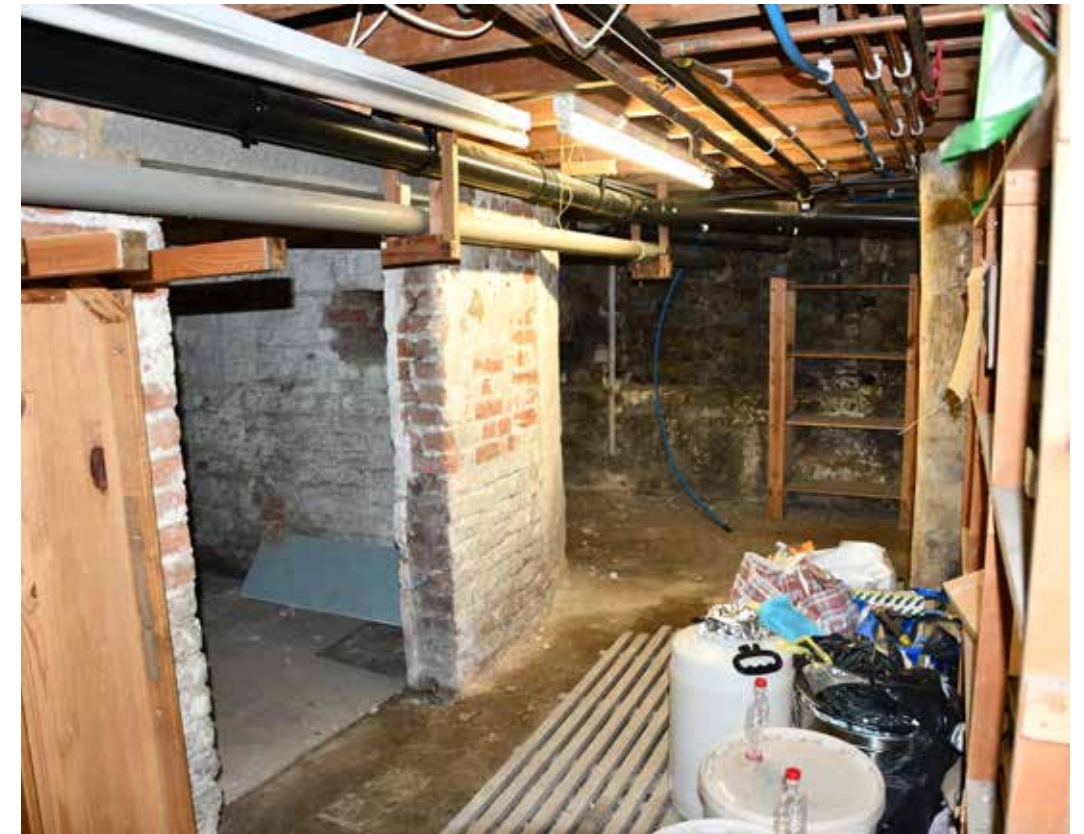
No. 808 Basement with fragments of historic fabric
