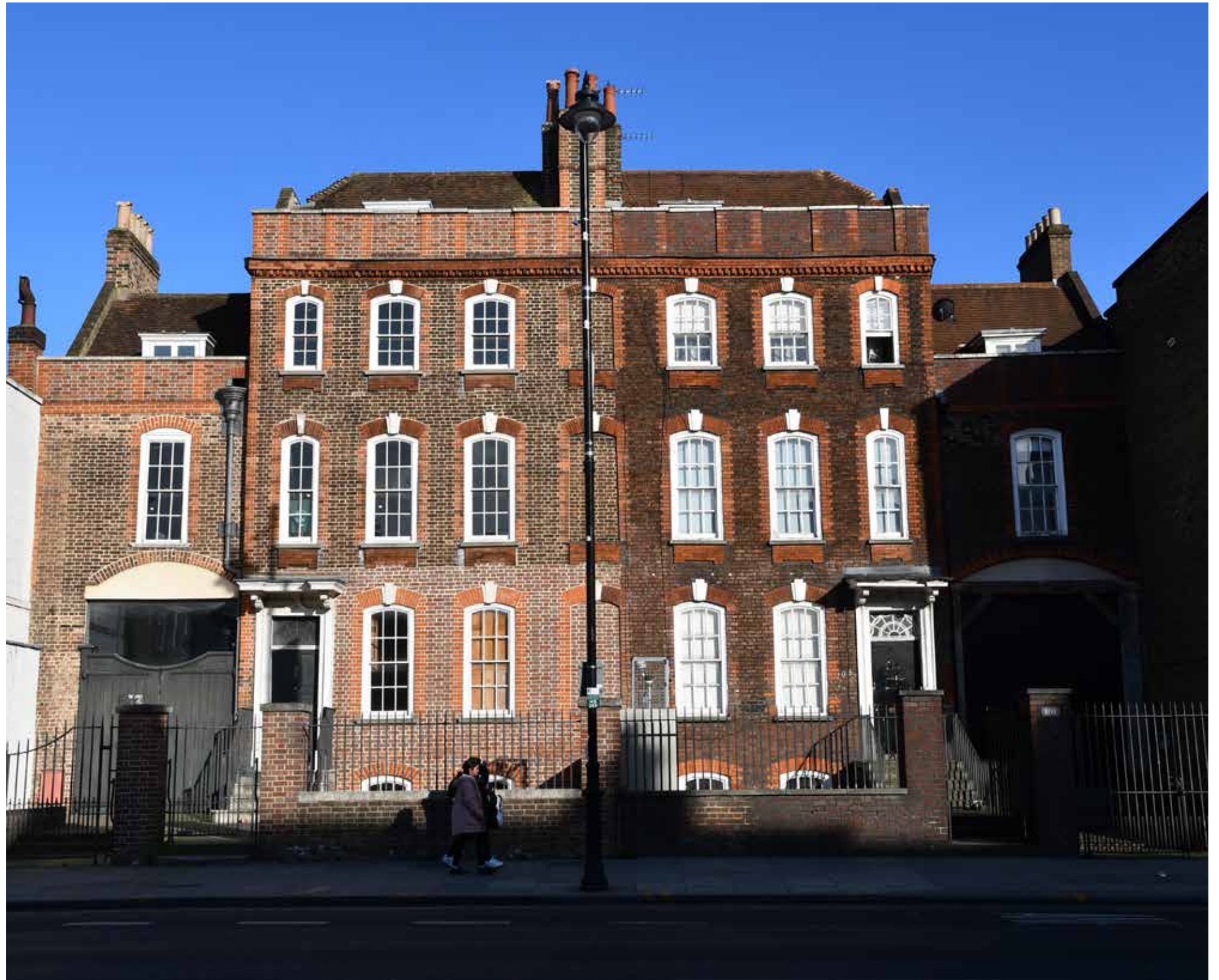
FIGURE 1. Street elevation of 808-810/812
