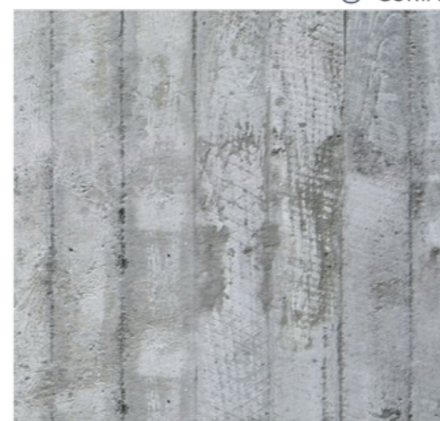
⑥ SHUTTERED CONCRETE
