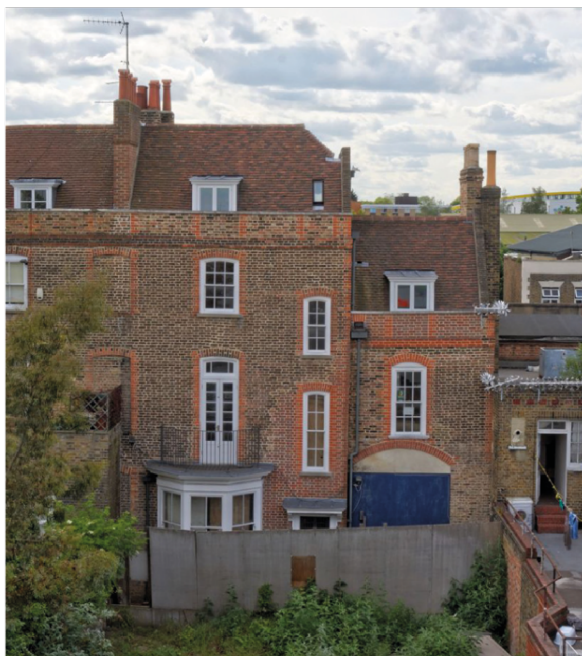
③ EXISTING REAR ELEVATION - STOCK BRICKWORK
