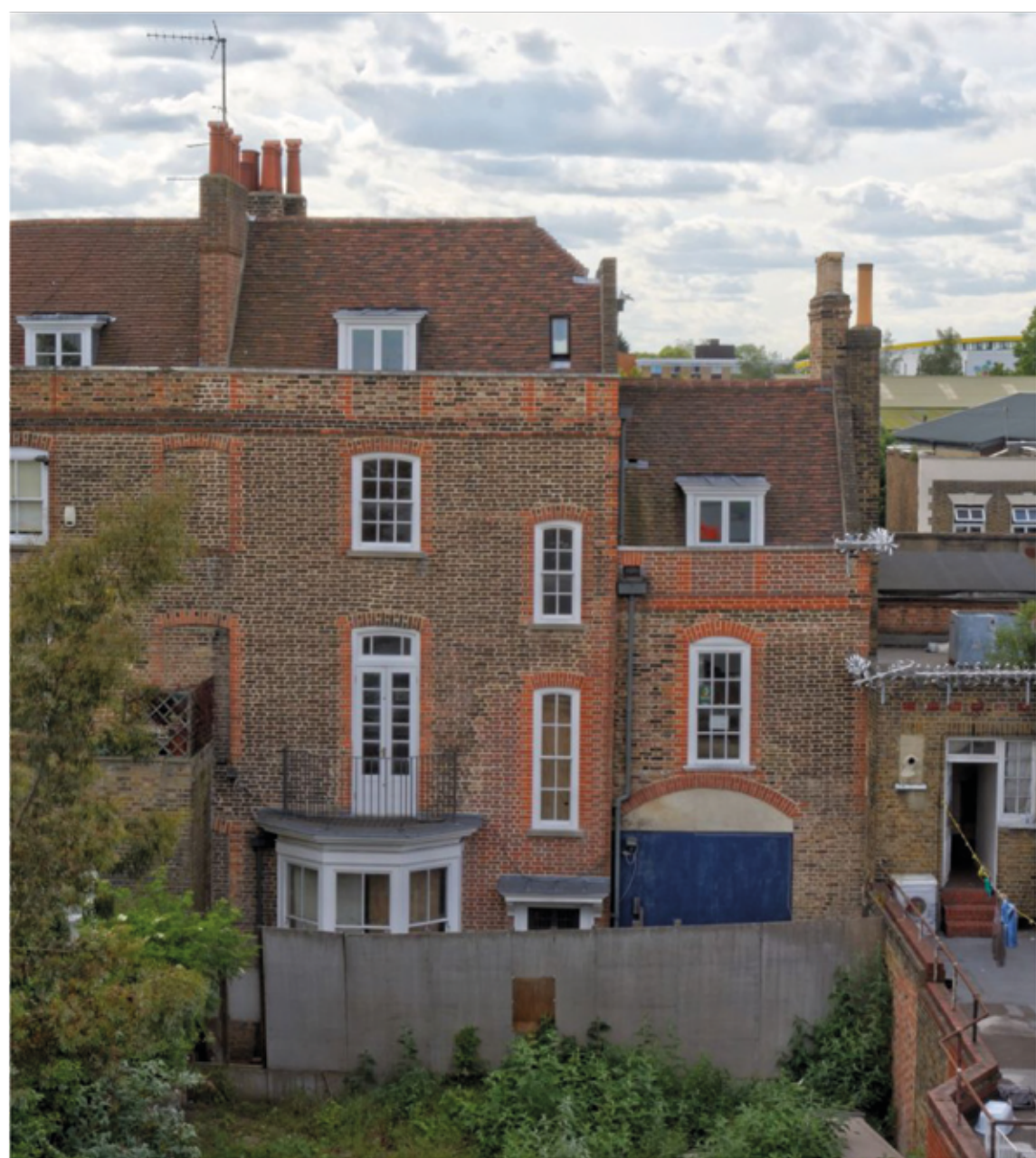
③ EXISTING REAR ELEVATION - STOCK BRICKWORK
