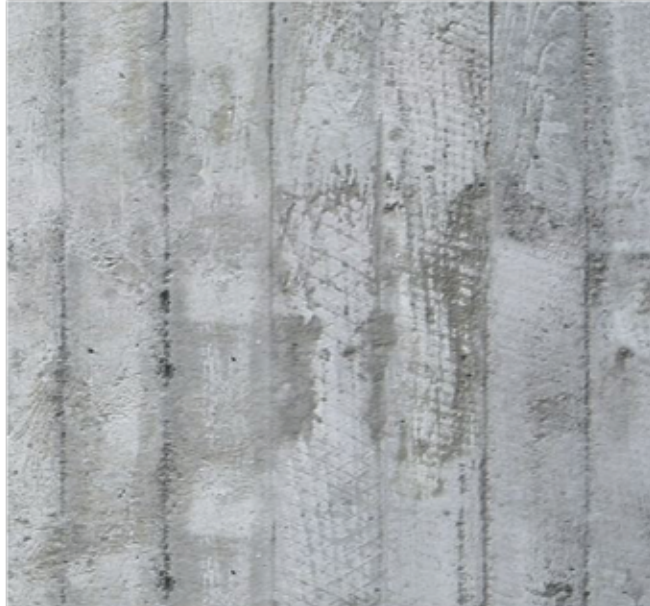
⑥ SHUTTERED CONCRETE
