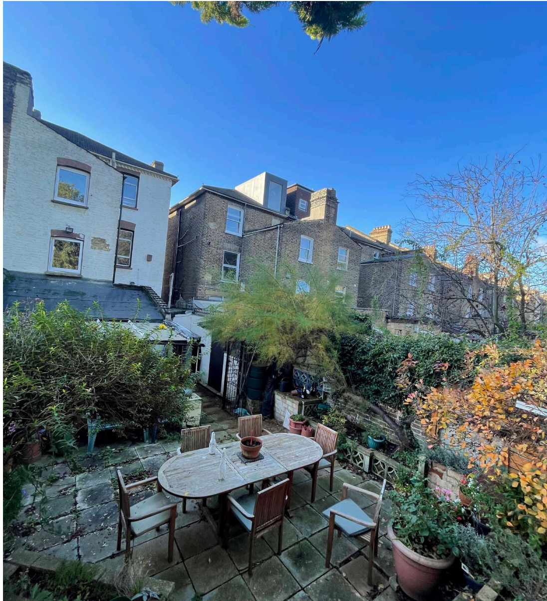
View of neighbours rear extension and rear dormer at 39 and 41 Florence Road
