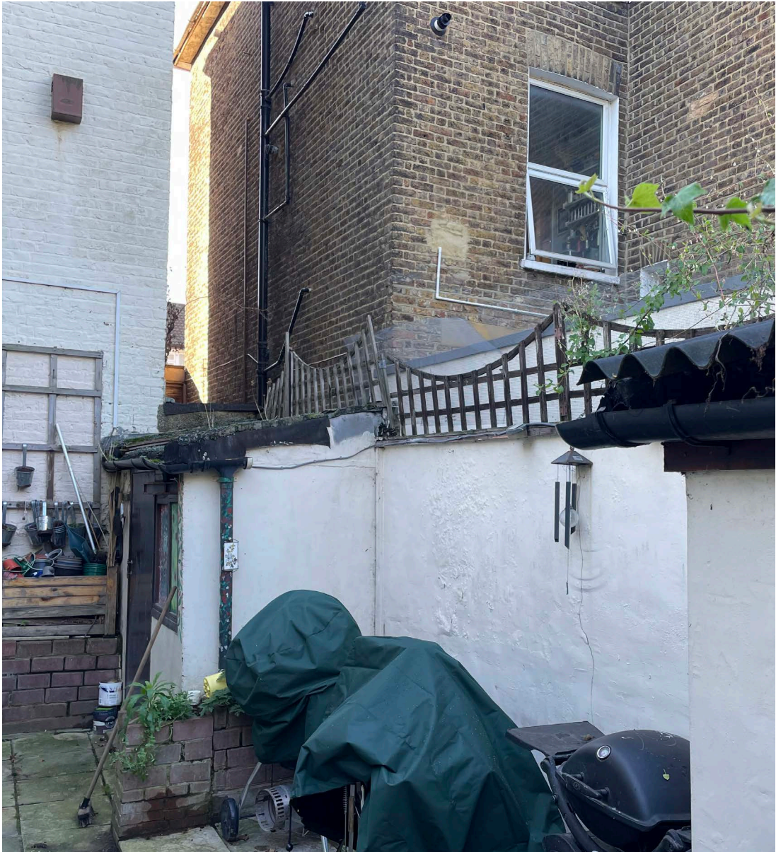
Existing side passage blocked by outbuilding
