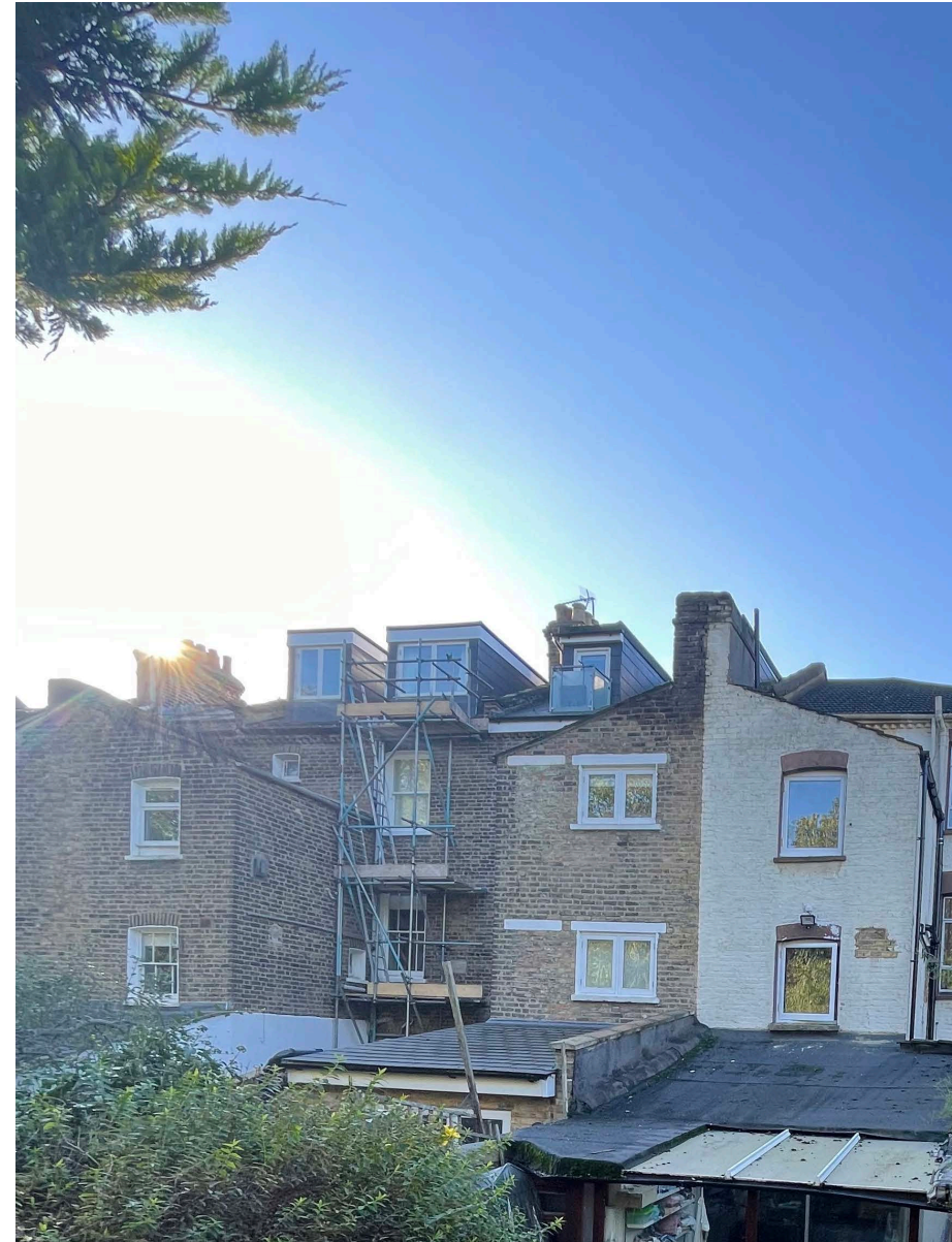
View of neighbours rear extension and rear dormer at 33 and 35 Florence Road
