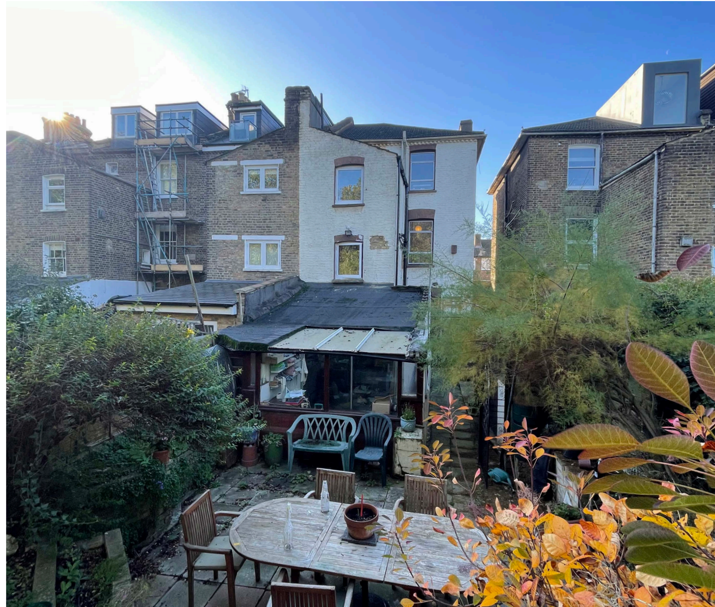
Rear elevation with existing extension and painted rear facade
