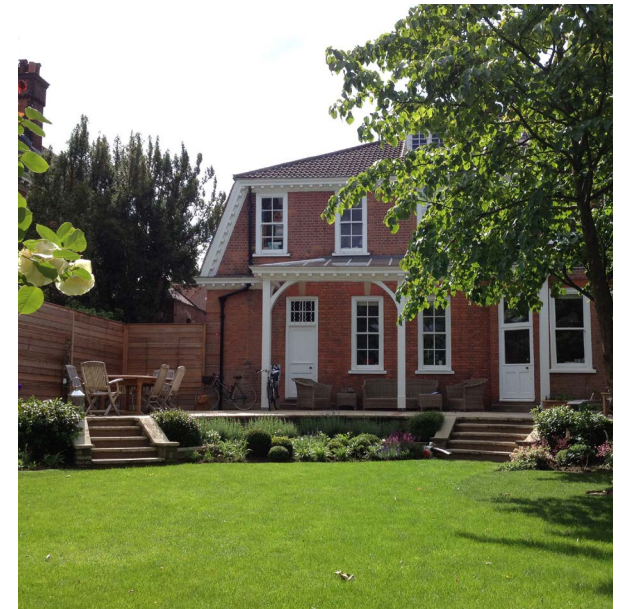
Figure 6 Rear elevation of the Listed Building as seen from the garden.
