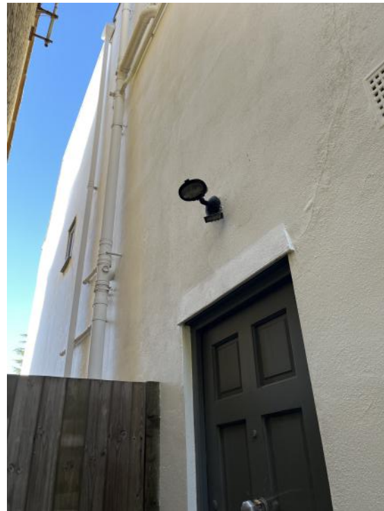
3. Side elevation and side access to first floor
