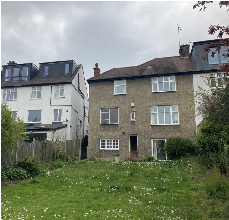
REAR ELEVATION - Showing no. 4 Creighton Avenue
