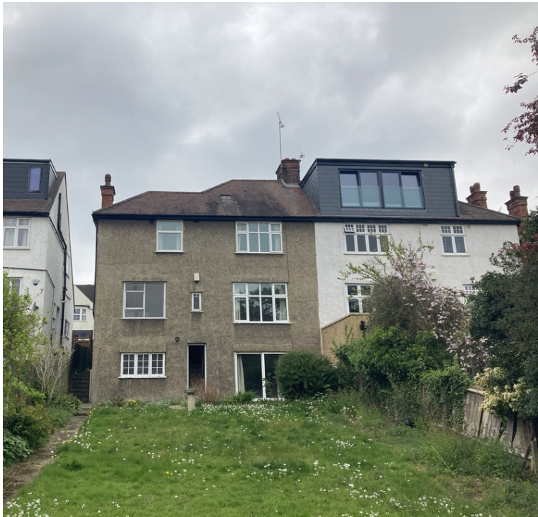
REAR ELEVATION - Showing no. 8 Creighton Avenue
