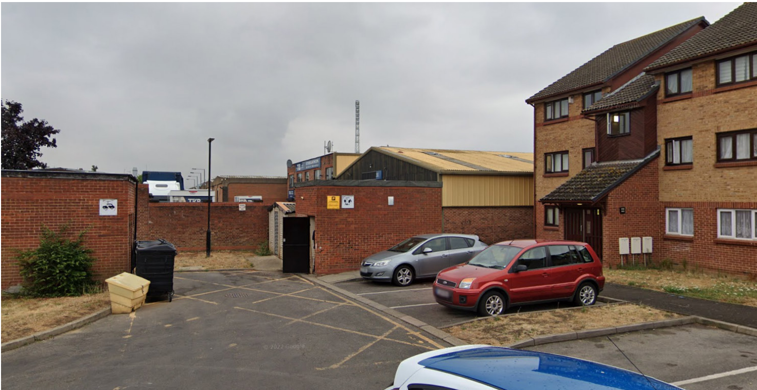
Local context: Rosebery Industrial Park
