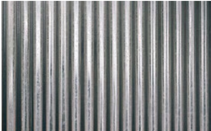
Existing materiality: Corrugated sheeting creates rhythm
