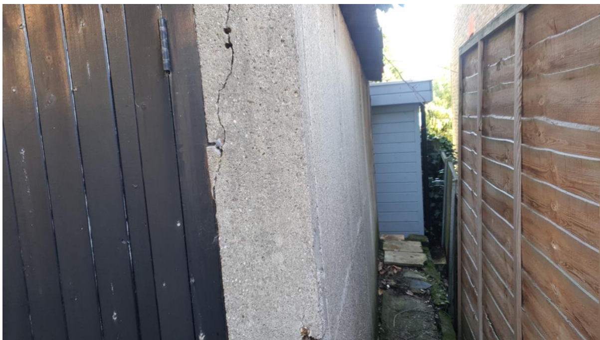
View to RHS of existing building
