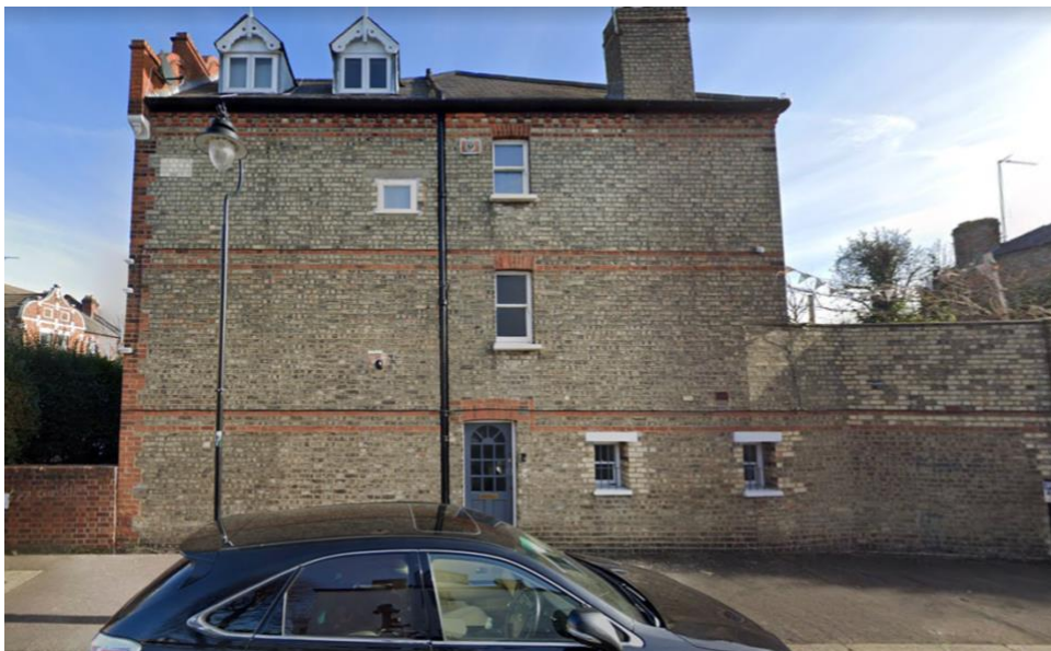
Side elevation of main property from Aubrey Road
