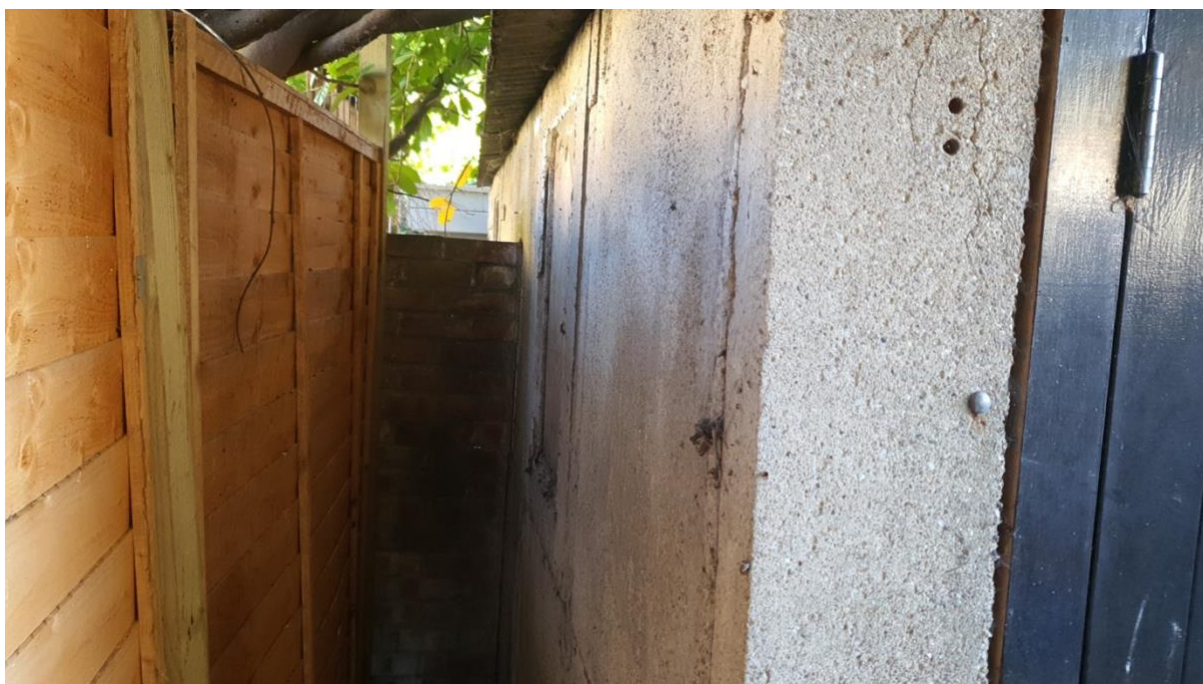
View to LHS of existing building
