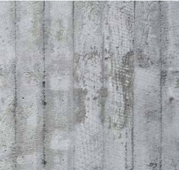
⑥ SHUTTERED CONCRETE
