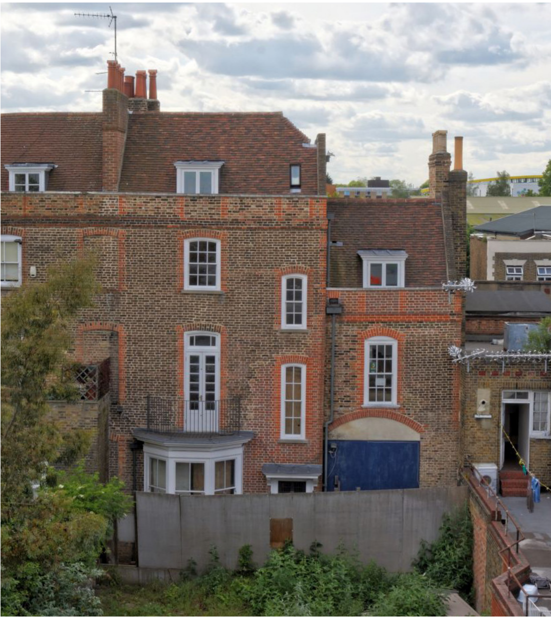
④ EXISTING REAR ELEVATION - STOCK BRICKWORK
