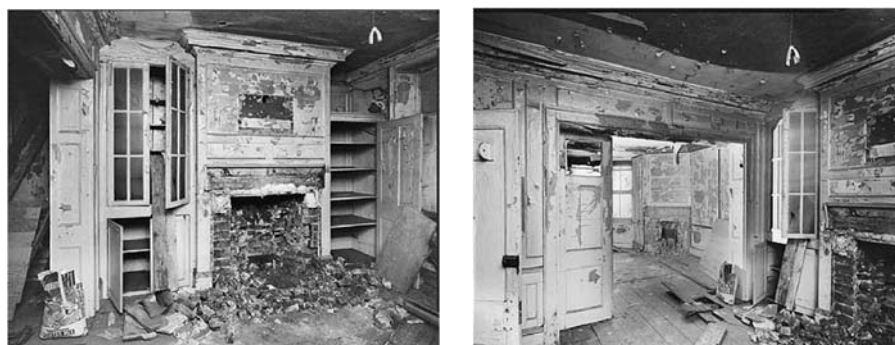
(above) 1991 RCHM record photographs of fireplace wall and view towards rear room.
