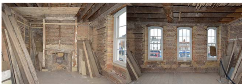
Existing after structural repairs and reinstatement of front windows
