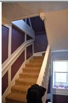
(Left) Stair SF-FF with original open balustrade and panelled partition. (Centre) Stair with original panelled partition, dado, cornice and pendant. (Right) Looking up to Second Floor
