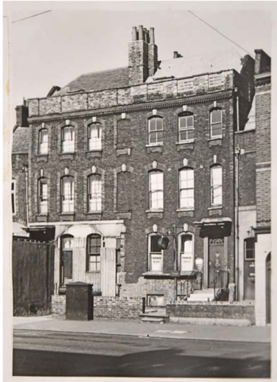
(Left) Figure 11. Undated photograph c1950, showing extensive damage and poorly matched brick repairs on the front elevation, likely to be the result of the WW2 bombing. The Confectioner's shop has been demolished, but the poorly matched brickwork and projecting bay at ground level of 808 has not yet been rendered.
