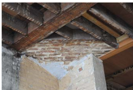
(Left) Underside of hearth above
