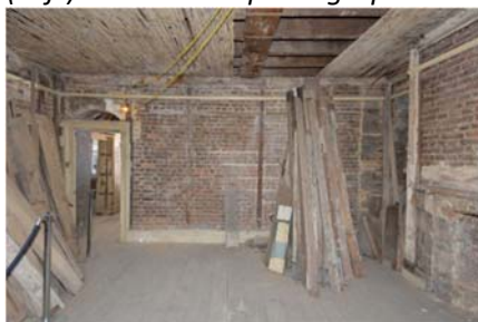
(Left) existing showing door head and ceiling after structural repairs (centre) wallpaper on fireplace wall
