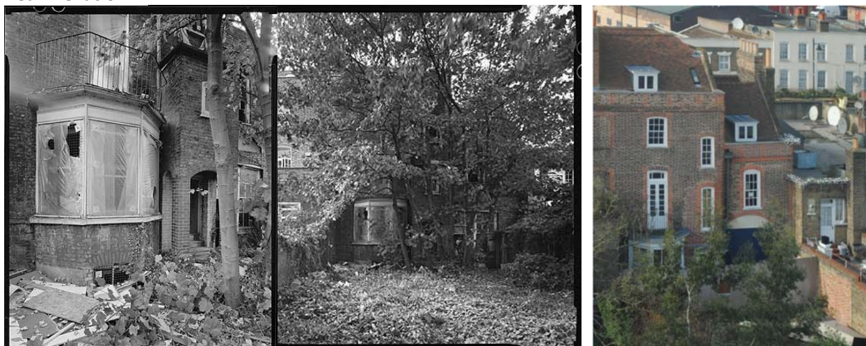
(Left and centre) 1991 RCHM photographs prior to C21 stabilisation and removal of extensions. (Right) Existing rear elevation including rebuilt bay, rear openings and boundary wall.
