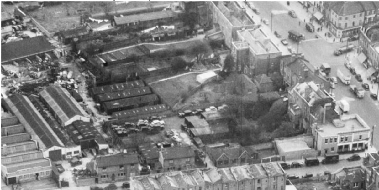
Figure 10 - Aerial View from North, 1961. This shows the rear of the houses with extensions. That at 808 is 3 storeys high, close to roof level of the Coach houses.
