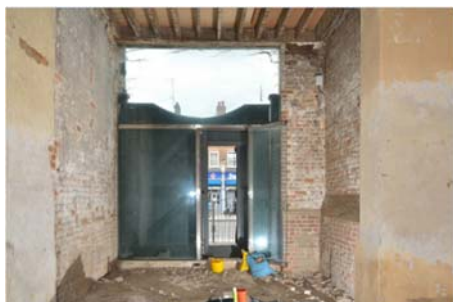
Looking towards front glass wall and gates
