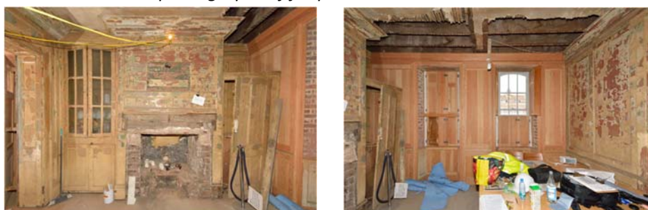
Fireplace, cupboards and section of replacement panelling and shutters on front wall from 2007-2009.
