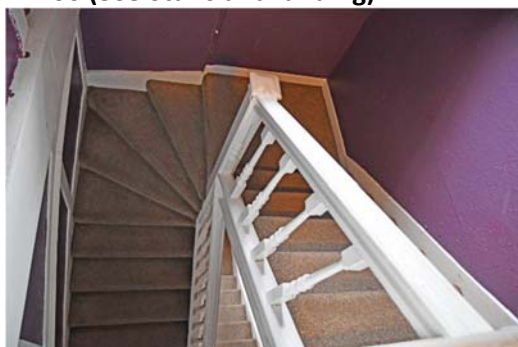
(Left) Stair SF-TF with original open balustrade. (Centre) Stair upper landing with C18 panelled partition
