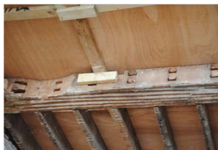
(right) large access hatch to be infilled
