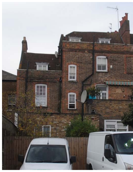
Figure 16: Rear of No 808 High Road - 2017
