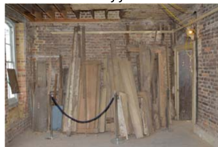
(Right) Typical extent of repairs
