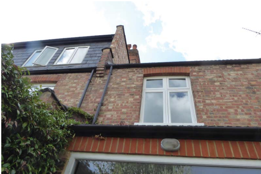
Rear elevation - with rear dormer at No. 40
