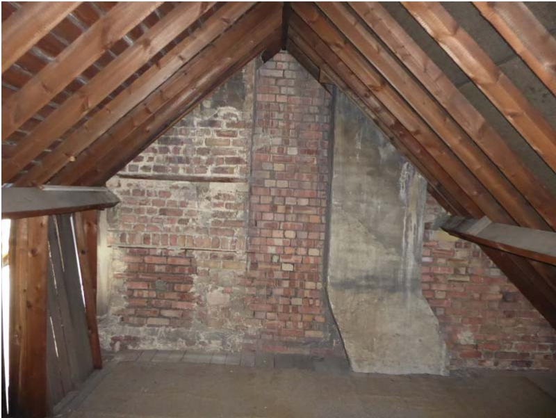
Loft space looking north
