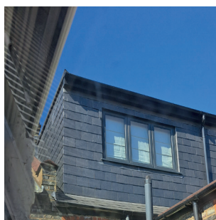
EXISTING DORMER AT 120 INDERWICK ROAD.
