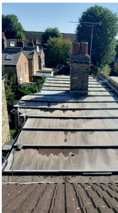
EXISTING FLAT ROOF
