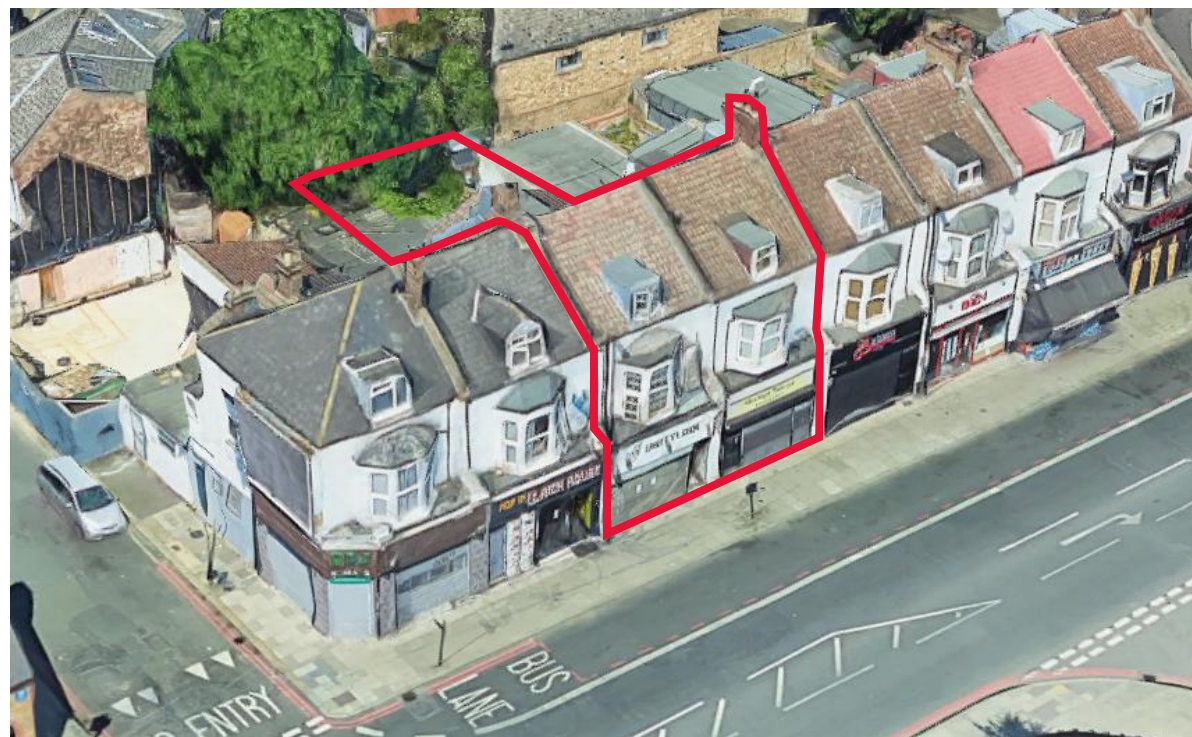
Existing building - Front
