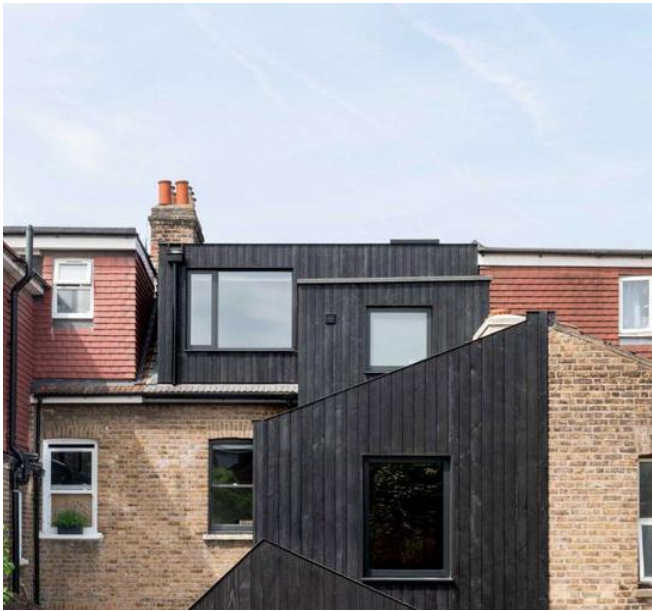
Black clad box dormer and first floor extension
