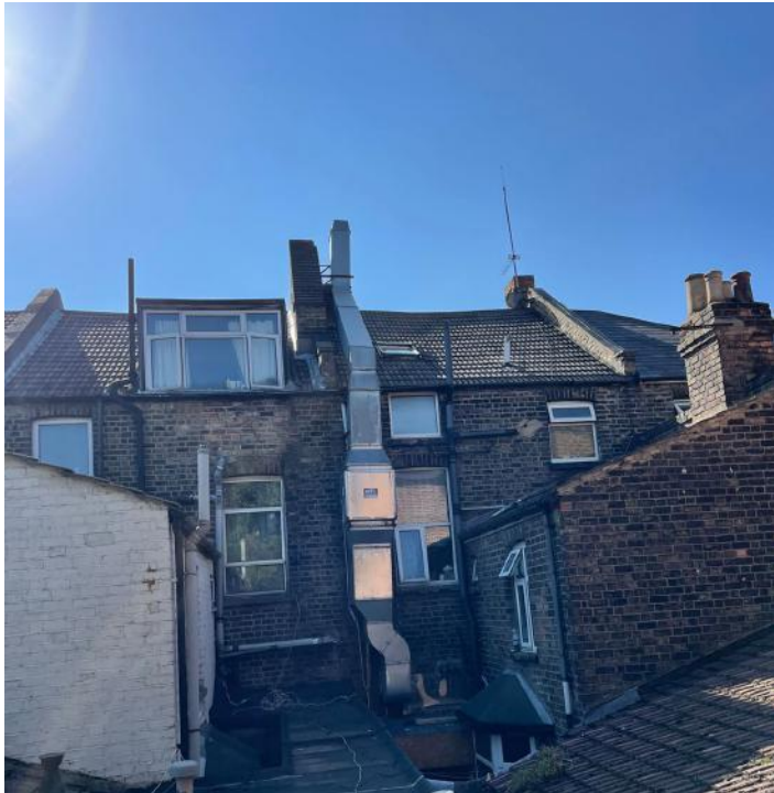
Rear elevation of 691 (ducting associated with 689)
