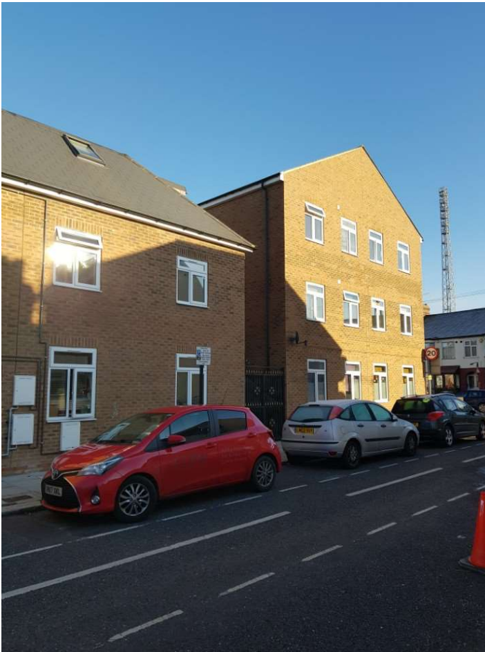
Position of mobile crane to lift steels on to top floor would be between red & silver cars.
