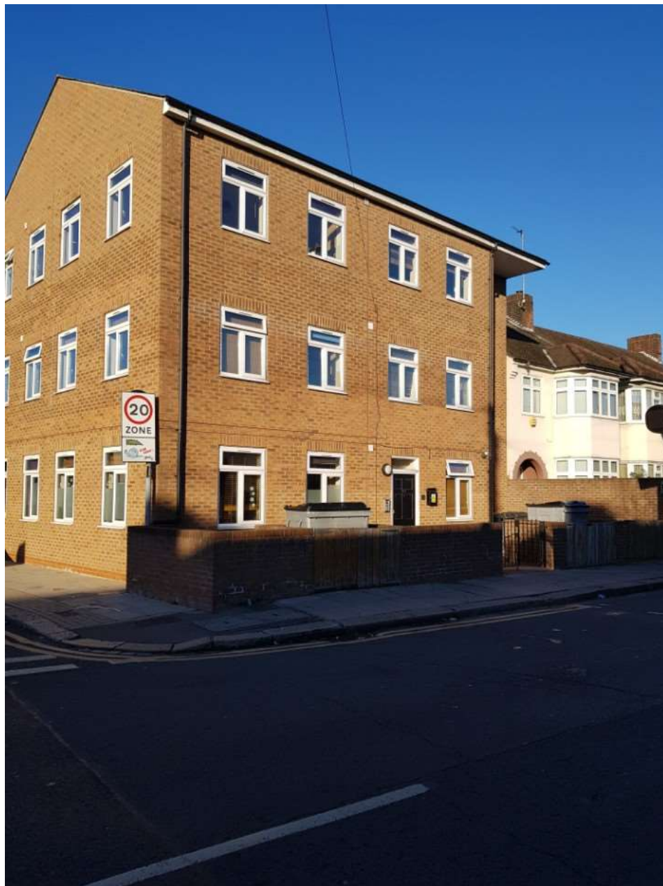
View of building on Shelbourne Rd – note that the telephone/data will be protected and if required re-located.
