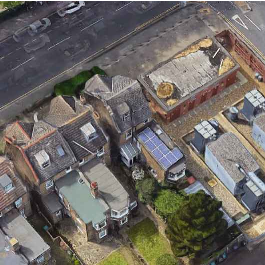
11 GREEN LANES PV panels on rear outrigger roof slope
