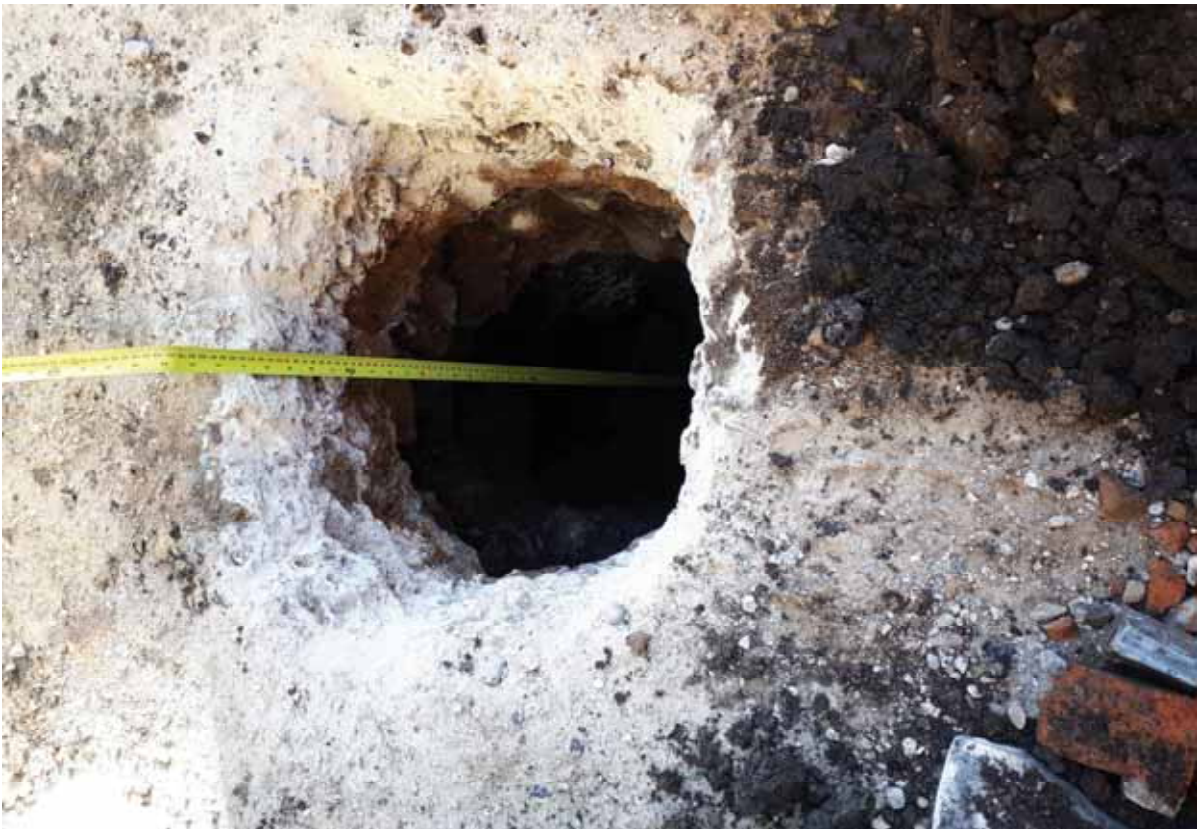
PH2 Inspection Pit 0.00m - 1.20m
