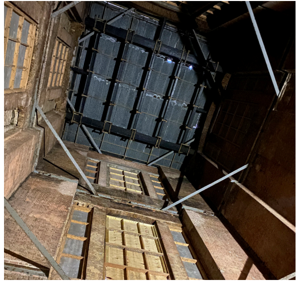
Figure 7: South West tower interior windows & roof
