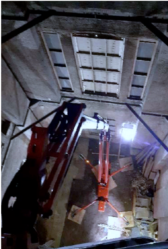
Figure 16: MEWP examines the internal roof structure
