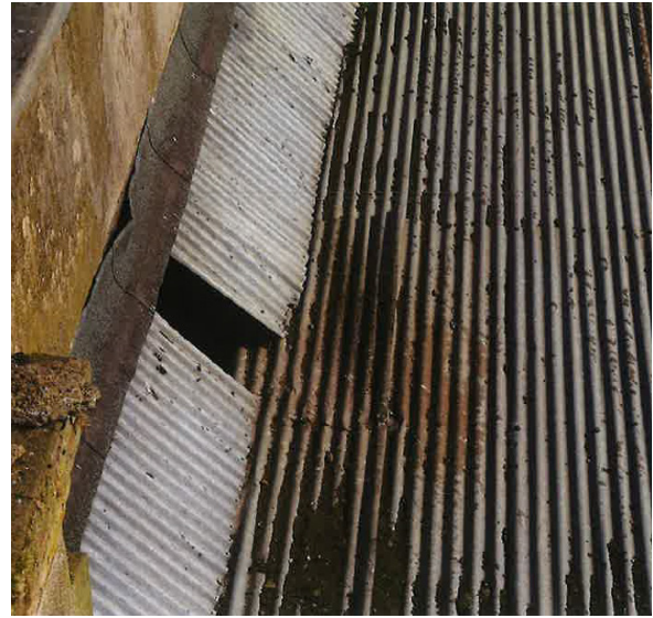
Figure 12: Corrugated iron roof
