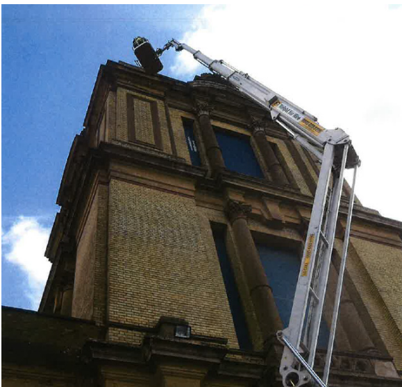
Figure 15: MEWP examines the roof of the tower
