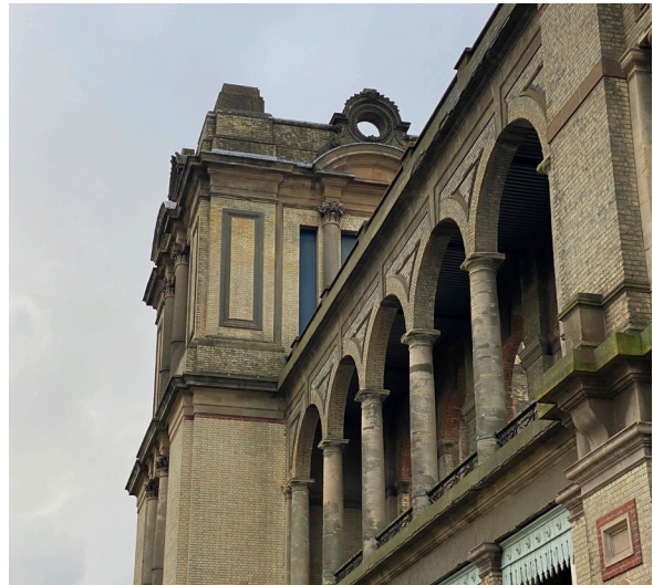
Figure 2: South elevation SW Tower
