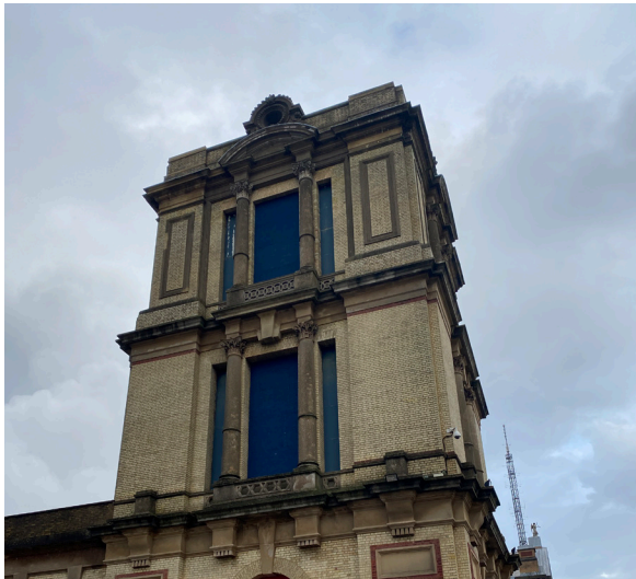
Figure 1: West elevation SW Tower
