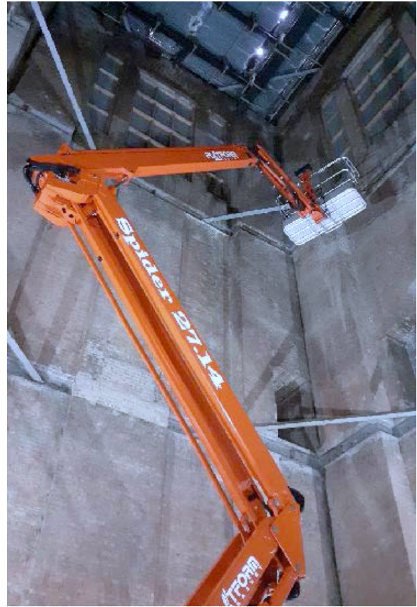
Figure 17: Internal void. MEWP examines the internal roof structure
