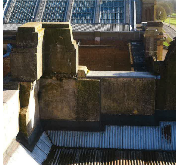
Figure 14: Corner junction to parapet
