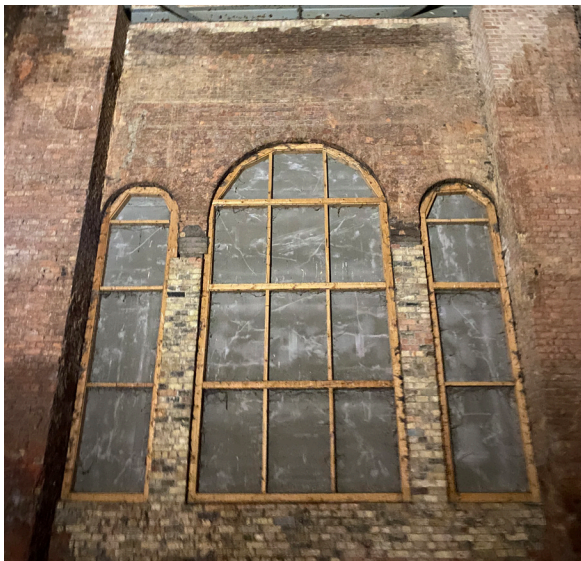
Figure 6: South West Tower interior windows
