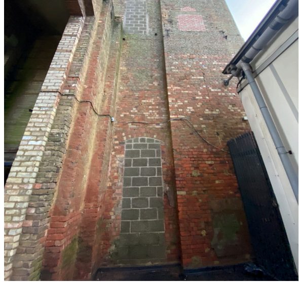
Figure 9: South West tower blockwork infills
