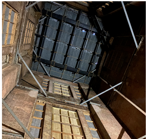
Figure 7: South West tower interior windows & roof
