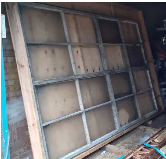
Figure 10: NE tower windows boxed up, to be repaired and reinstated in the SW tower
