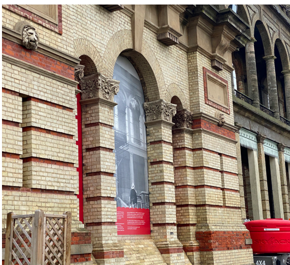
Figure 5: South elevation SW Tower
