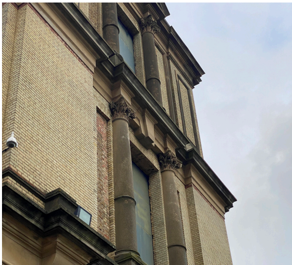
Figure 3: South elevation SW Tower
