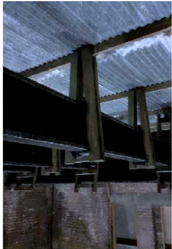
Figure 19: Cast Iron beam detail with 'A' frame timber roof structure and corrugated iron roof
