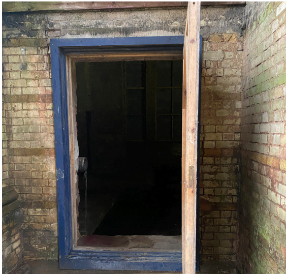
Figure 8: South West tower entrance
