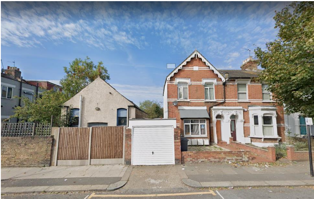
Existing street view
