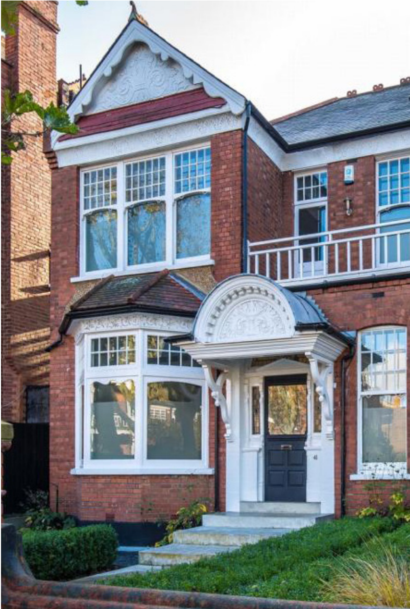
EXISTING FRONT ELEVATION - BAY WINDOW AND ENTRANCE
