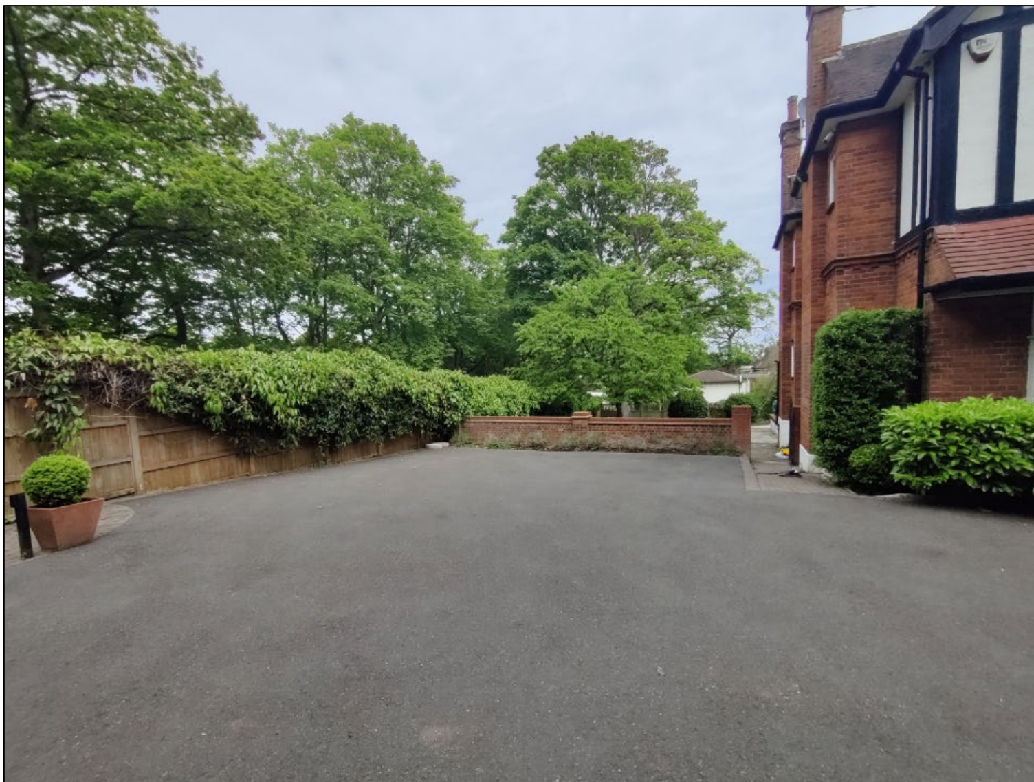
Photograph 2: Existing hard standing within site
