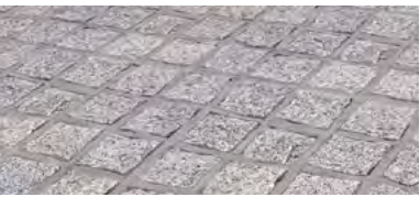
Sawn granite setts to thresholds
