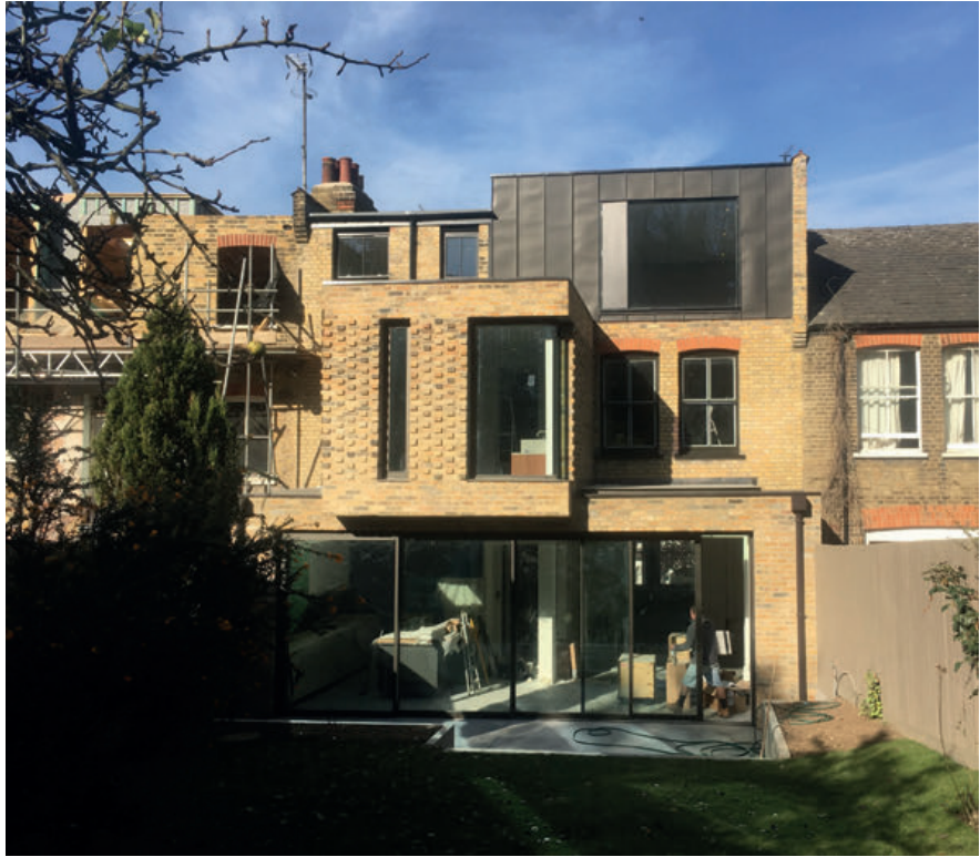
Dukes Avenue, N10 completed by MCA. Ref: HGY/2017/1542 30/06/2017
