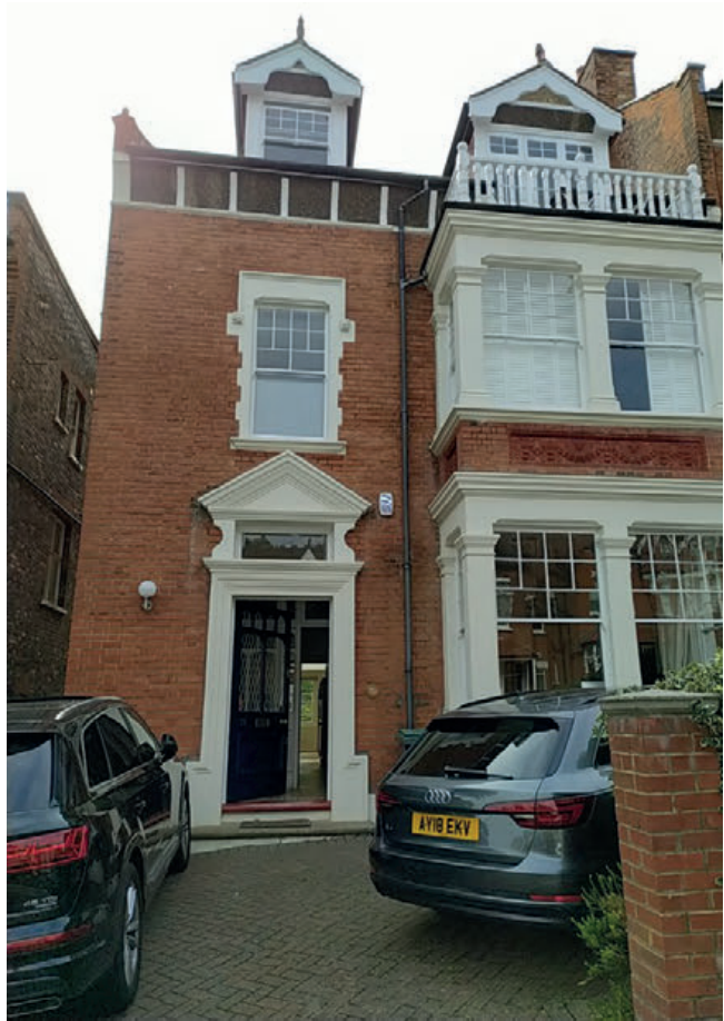
View from Southwood Avenue of the existing front elevation and hardstanding to the driveway.
