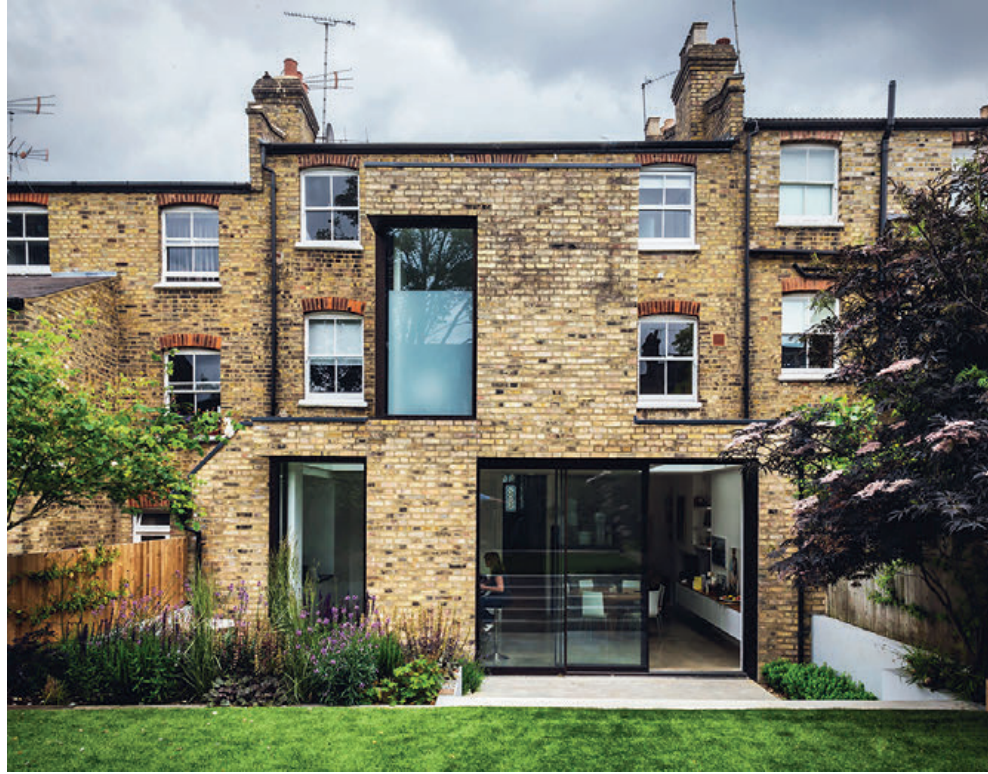
Nelson Road, N8 completed by MCA. Ref: HGY/2015/2090 11/09/2015
