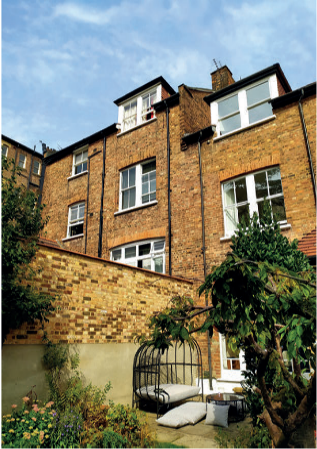
View of the existing retaining wall to the boundary with No.41
