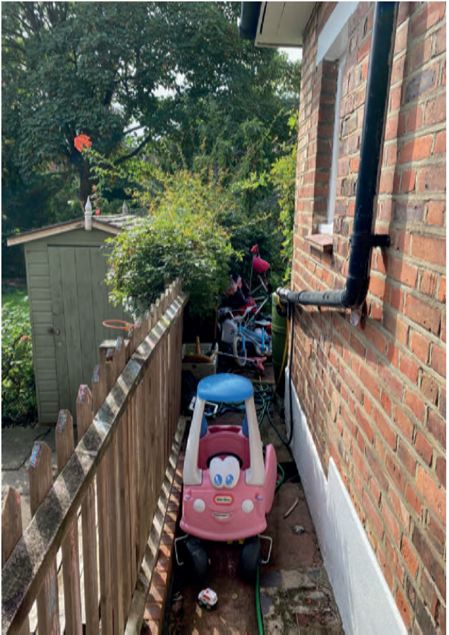
View of the existing boundary condition with No.37 including the existing window on the side elevation of the existing rear extension.
