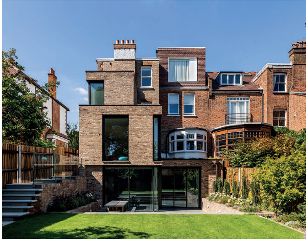
3 Southwood Lawn Road, N6- 3 storey rear projection extension completed by MCA. Ref: HGY/2016/1175
