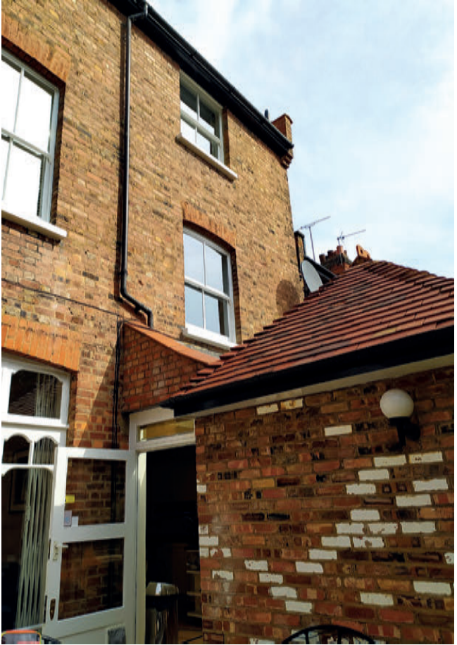
View of the roof profile of the existing non-original rear extension.
