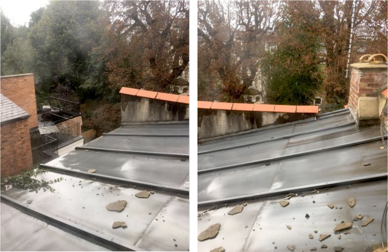
Photograph taken from rear of proposed terrace indicating the view and visual cut-off due to the parapet at the end of the existing roof
