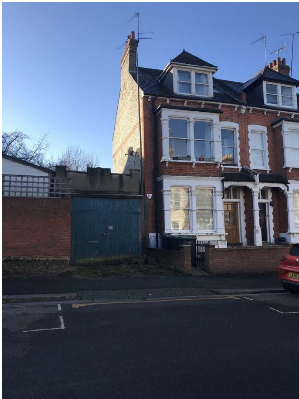
Figure 3. Photograph of garage site and no. 1 Ferrestone Road (above).
