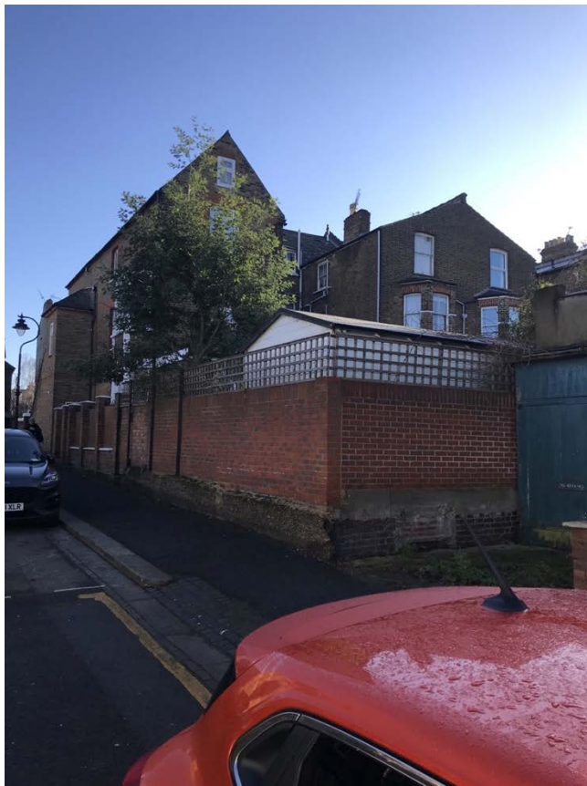
Figure 6. Part-view of the garage site with nos. 16 and 17 Church Lane (above).
