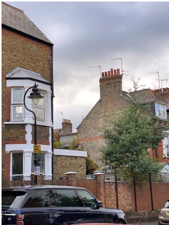
Figure 4. Oblique view of site with part of no. 16 Church Lane and gable end of no. 1 Ferrestone Road with the brick diamond and decorative banding (above).
