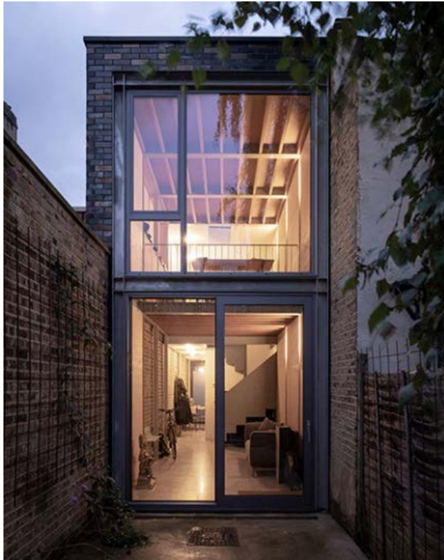
Figure 9. Slot House by Sandy Rendel Architects (above).
