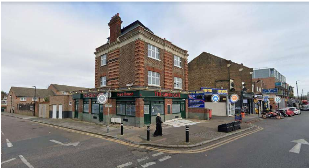
Street view image showing the existing (proposed) roof
