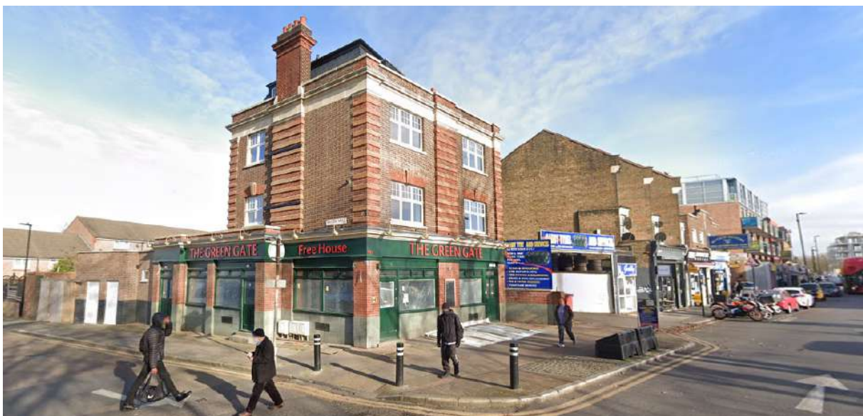
Current public house (2014 and 2022 photo showing the mansard roof)
