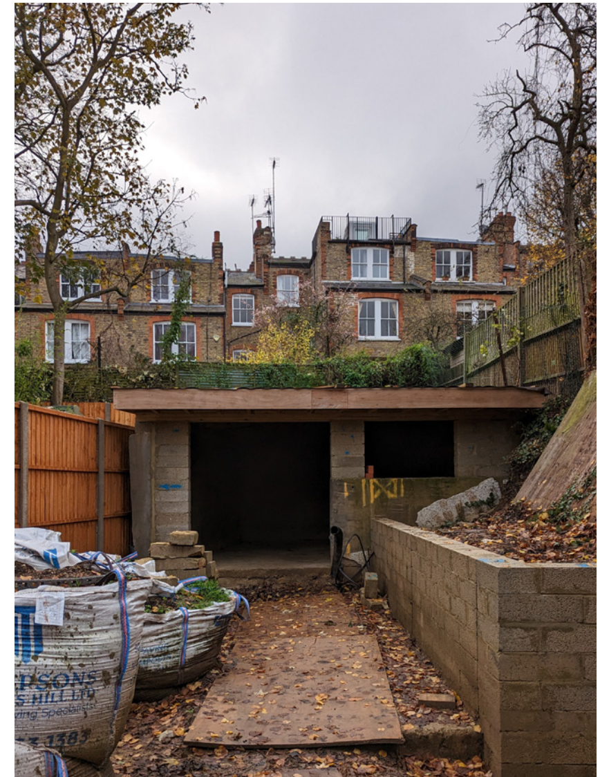
Fig. 07: Photo of rear garden November 2022. Note position of retaining wall in same position and raised.
