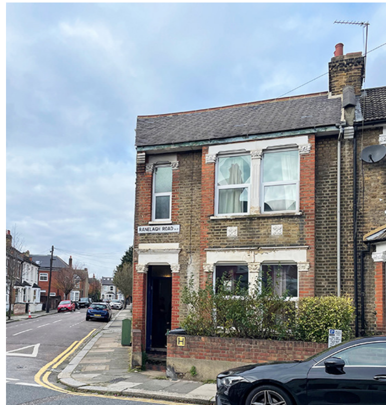
View of front of no. 33 Ranelagh Road
