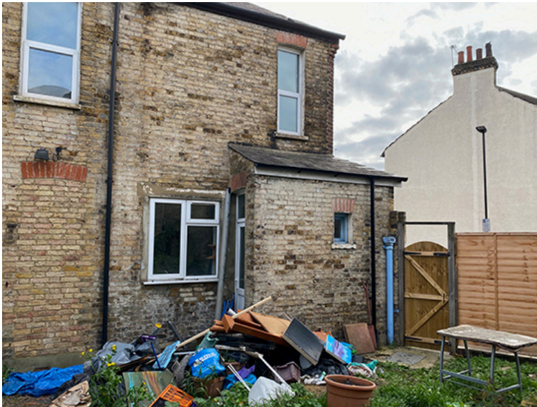
Rear elevation showing the existing shed
