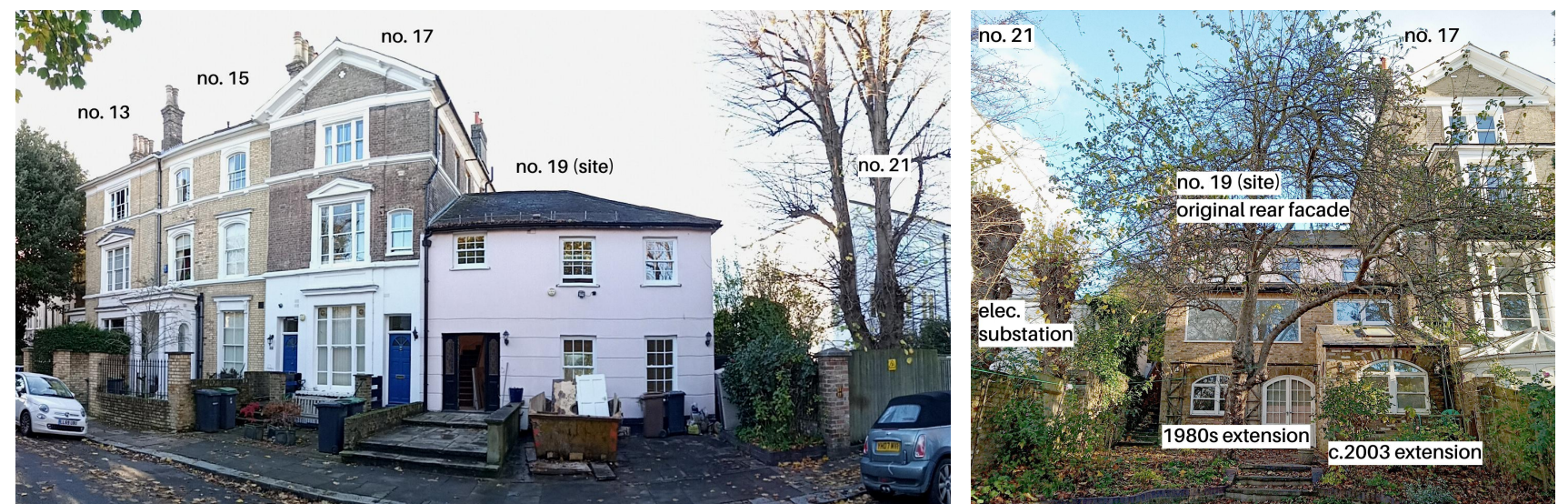
Site Photographs (Nov 2022) showing front elevation along North Grove (lower left) and rear elevation on sloping site (lower right), with original facades in pale pink stucco and rear extensions in London stock brick
