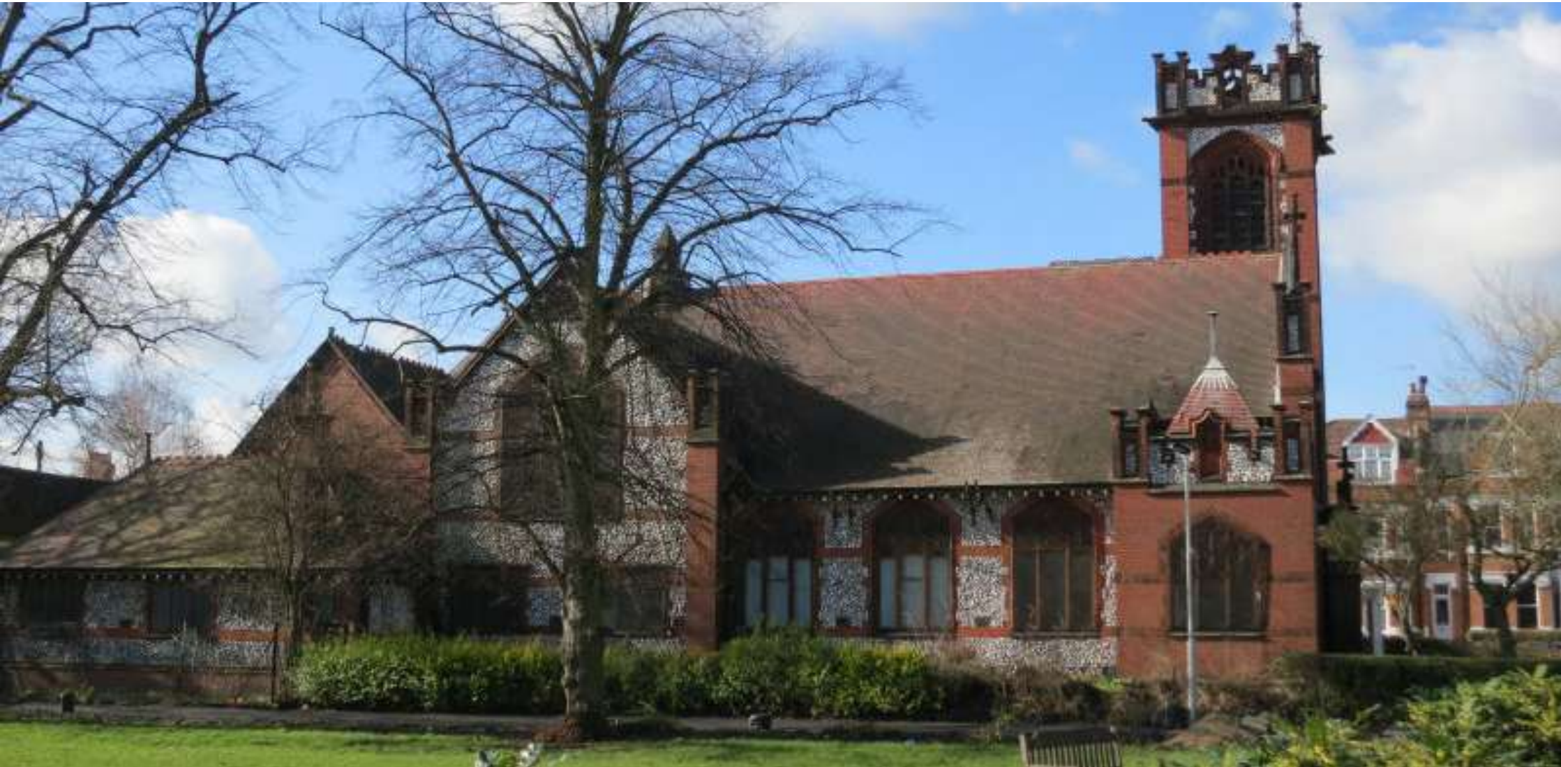
Existing building on Site
