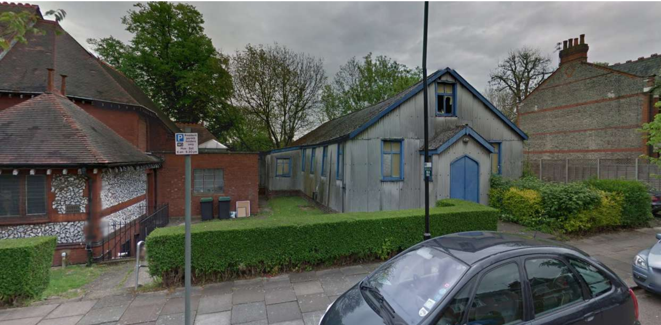
Existing tin tabernacle on Site
