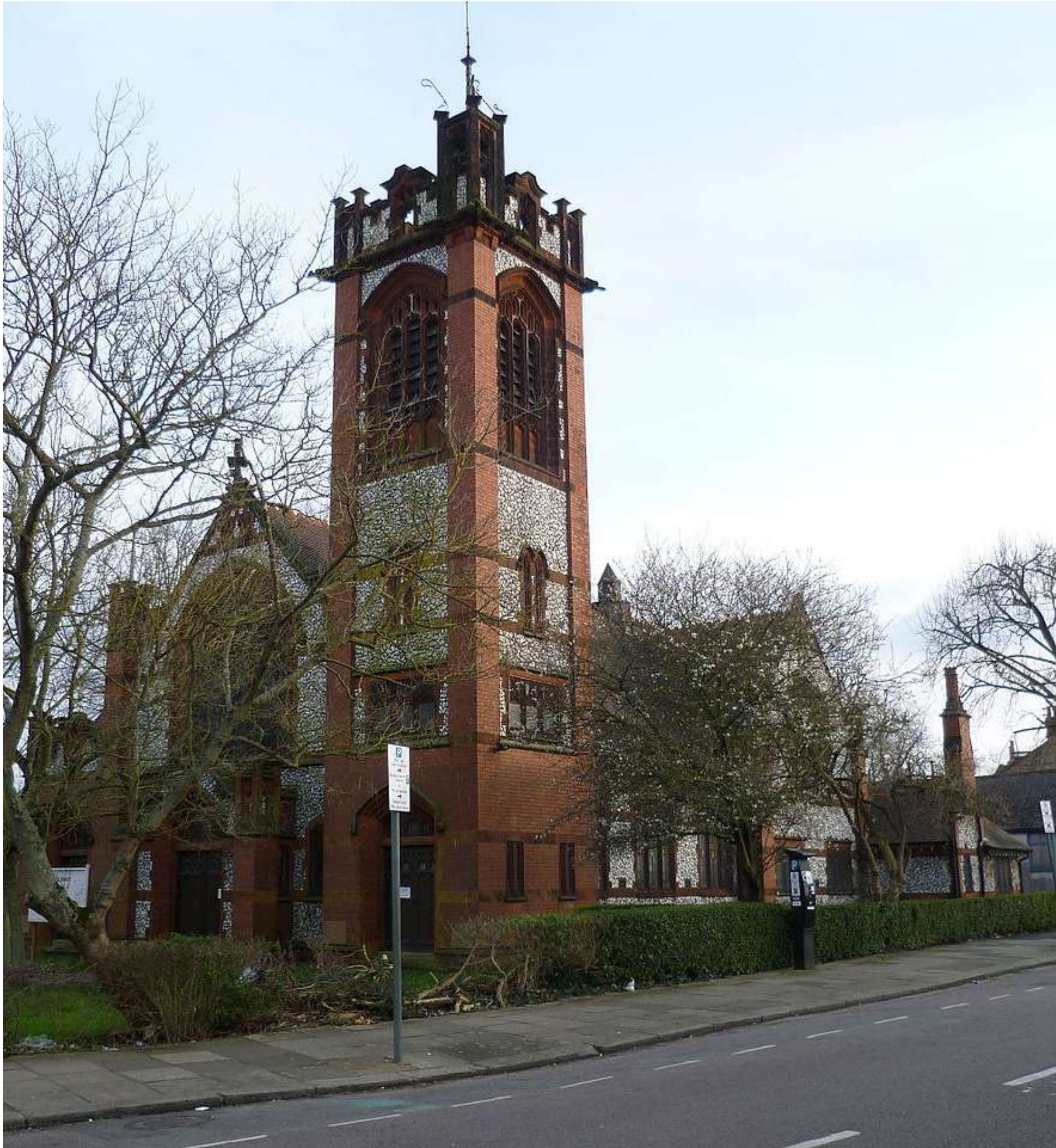
Existing building on Site
