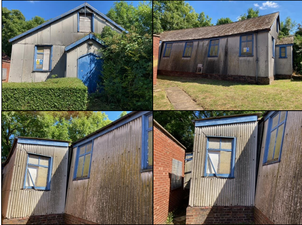
Photographs 9 - 12: Church Hall
