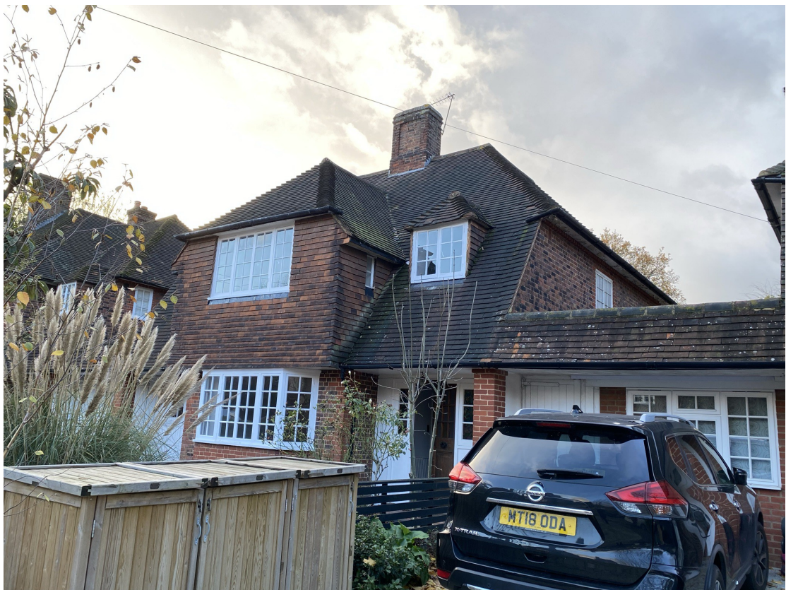
View of house from northeast, showing part of the north flank elevation
