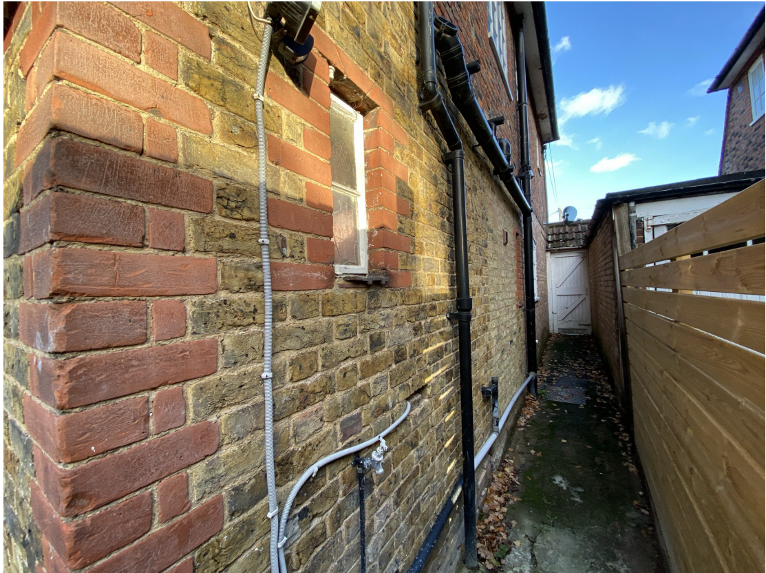
Side passageway to south of building
