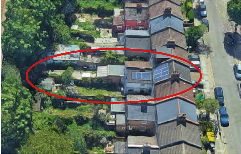
Aerial view from North
