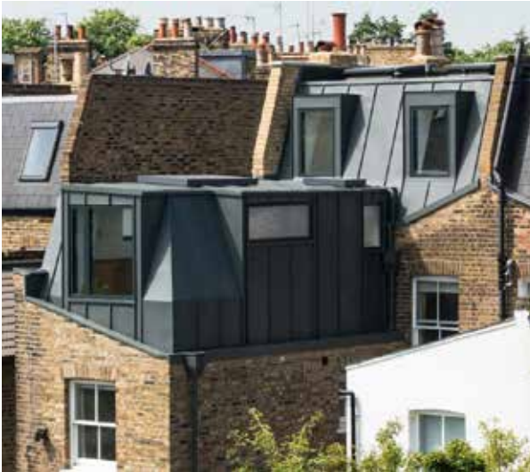
Example of dormers with metal cladding
