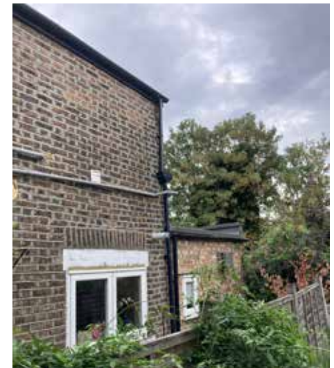
Rear extension to No. 45
