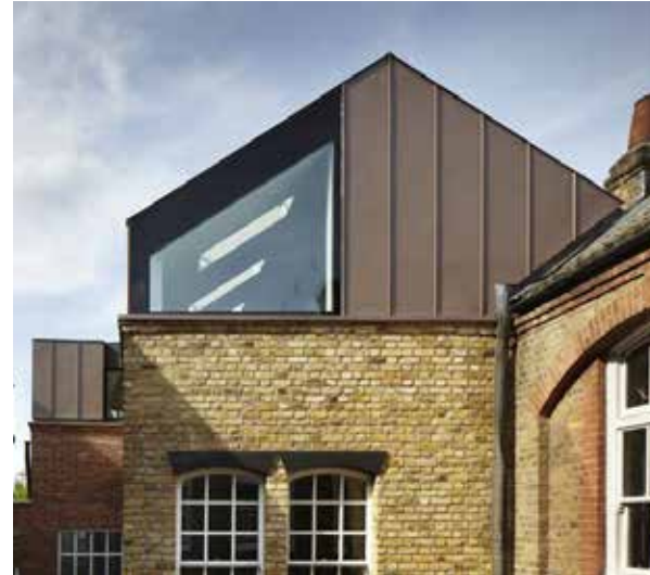
Example of roof extension with metal cladding
