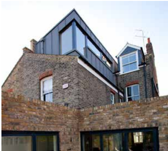
Example of roof extension with metal cladding
