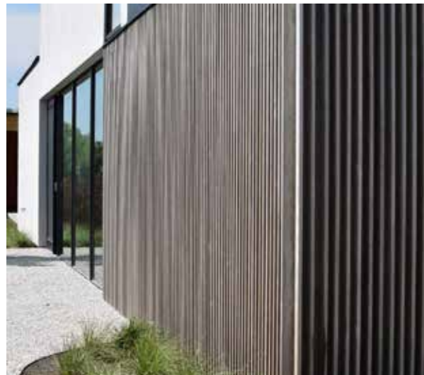
Weathered timber cladding
