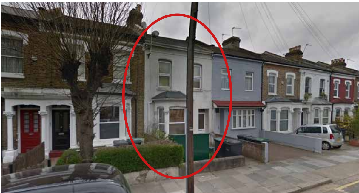
Front elevation view from Google Streetview - 2016
