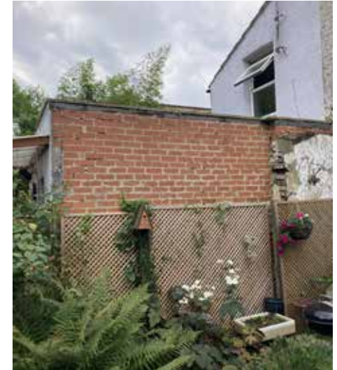
Rear extension to No. 41
