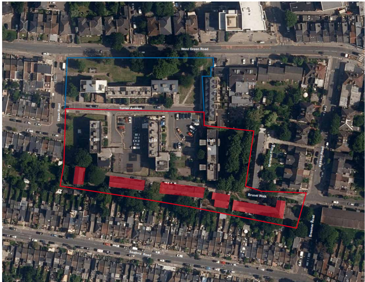
Aerial view of site
