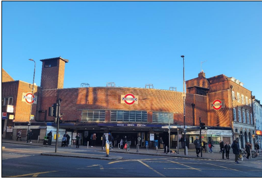
Photo 3. The Grade II Listed Wood Green Underground Station from the south west corner of the junction
