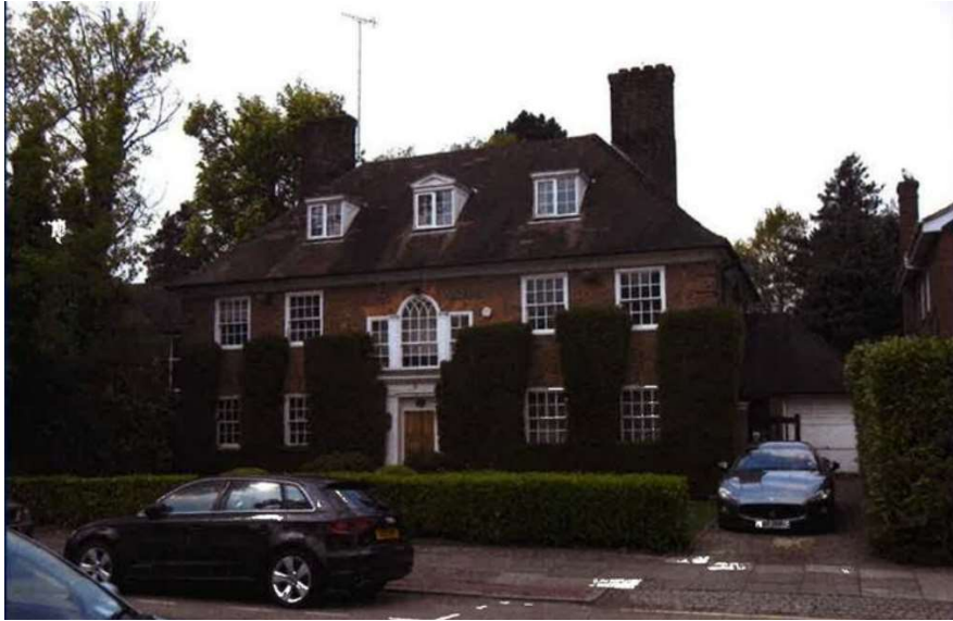
Figure 3.15: Photograph of No.21 Sheldon Avenue dated c.2015, prior to its redevelopment (including façade retention)
