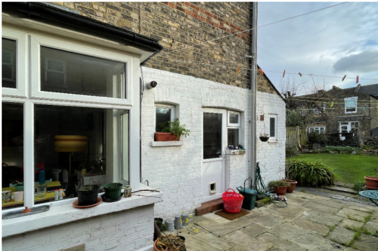
View 1 Looking towards the garden
