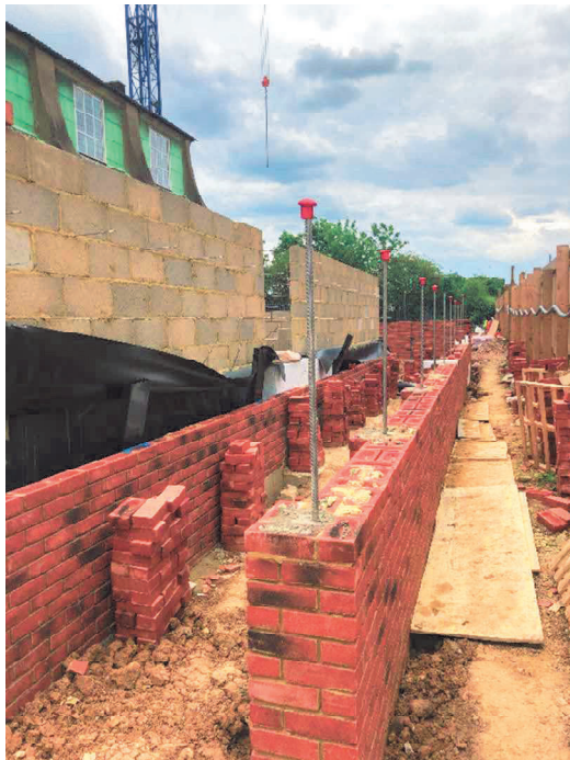
Retaining Wall H3 16/06/20
